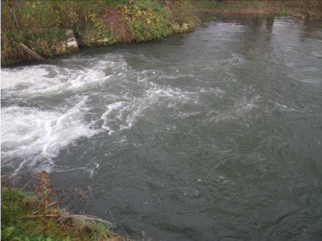
Photo 2. Top weir on the Craven provides the head of water for the mill/carrier channel.
