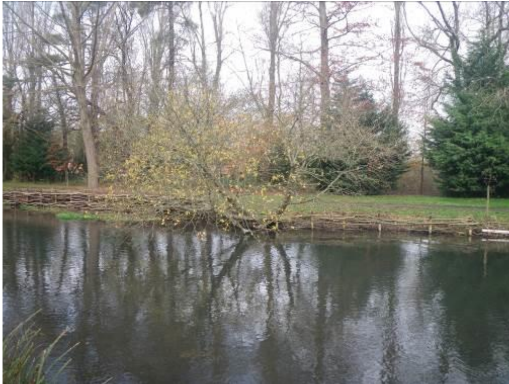
Photo 5. Left bank erosion repairs.
