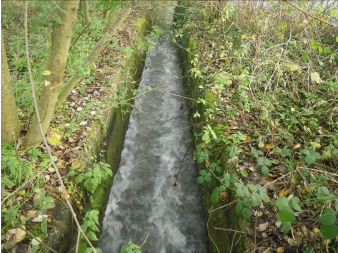
Photo 3. Fish pass installed by the EA.
