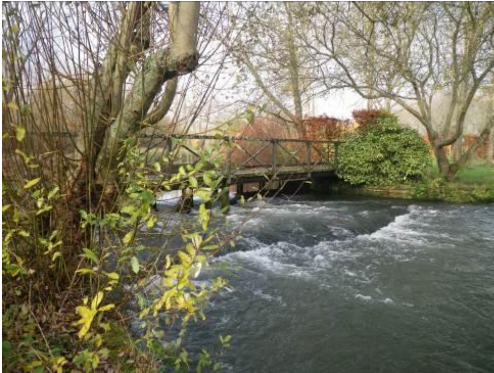
Photo 6. Removing all the hatches and cutting a 3-4 m wide notch in the weir invert would significantly improve habitat quality in the reach above.
