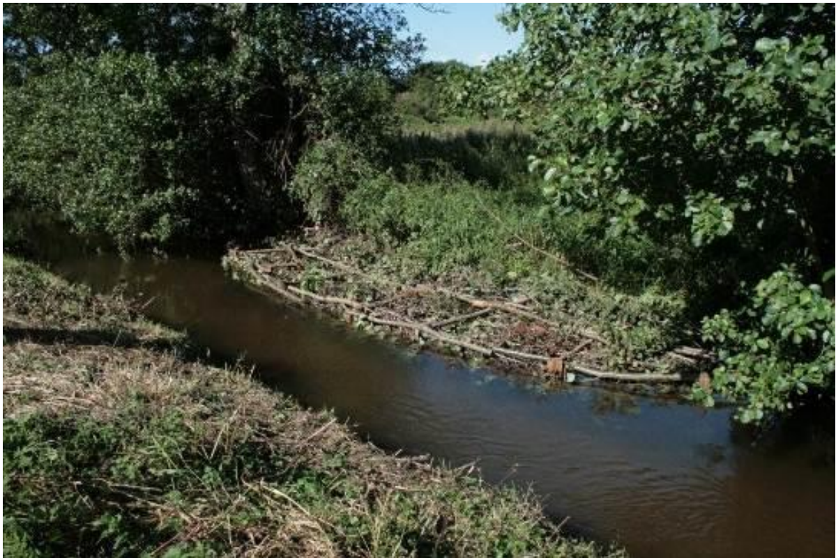
Photos 9 and 10. Typical examples of brushwood berms
