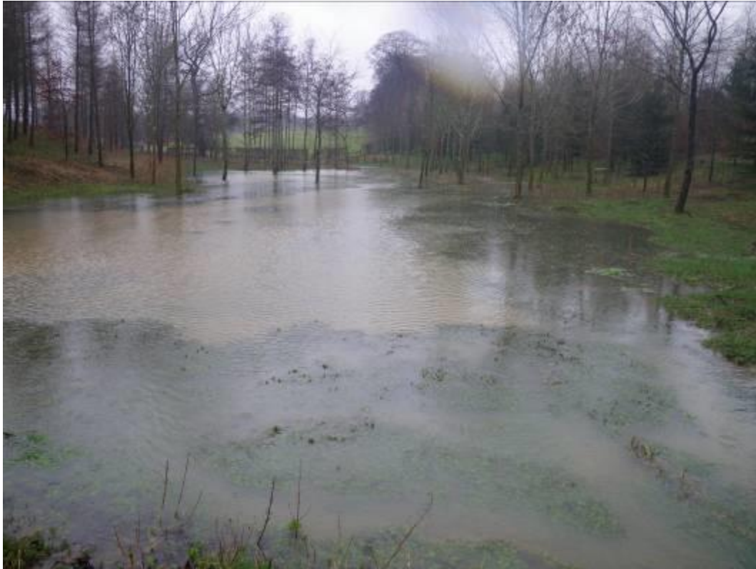
Figure 3. Local flooding exacerbated by the partial blocking of the culvert.
