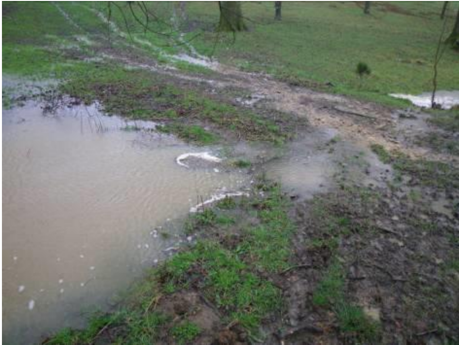
Figure 5 partially blocked culvert causing upstream flooding and sediment deposition.
