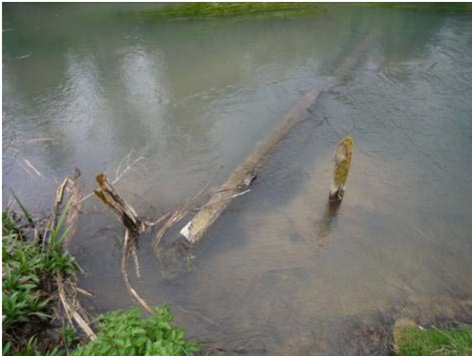
One half of a downstream "V" deflector. Increased water velocities are being directed towards the bank, gradually making the channel wider rather than scouring a central run.
