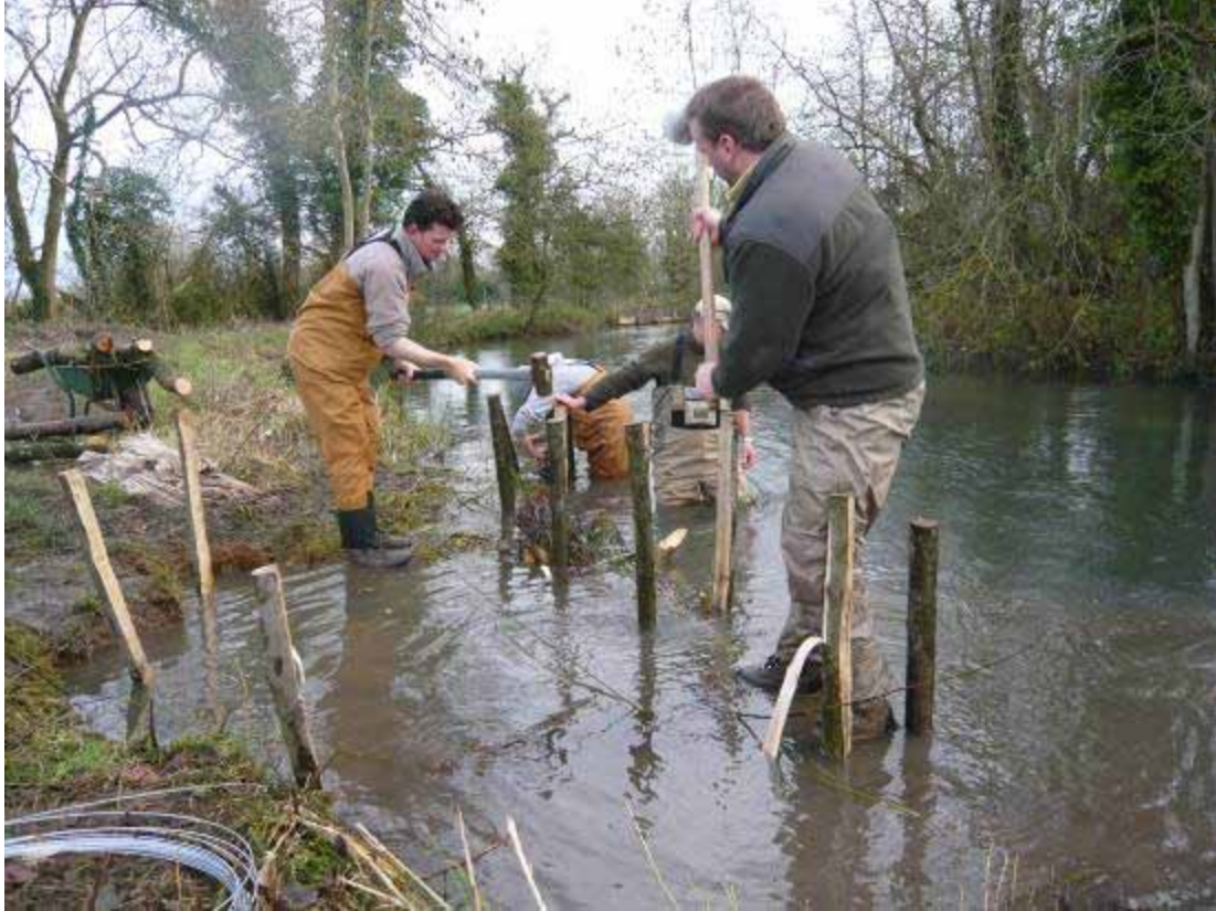
Members of the Bull fishing group get to work combating marginal erosion during the WTT Practical Visit in November 2008
