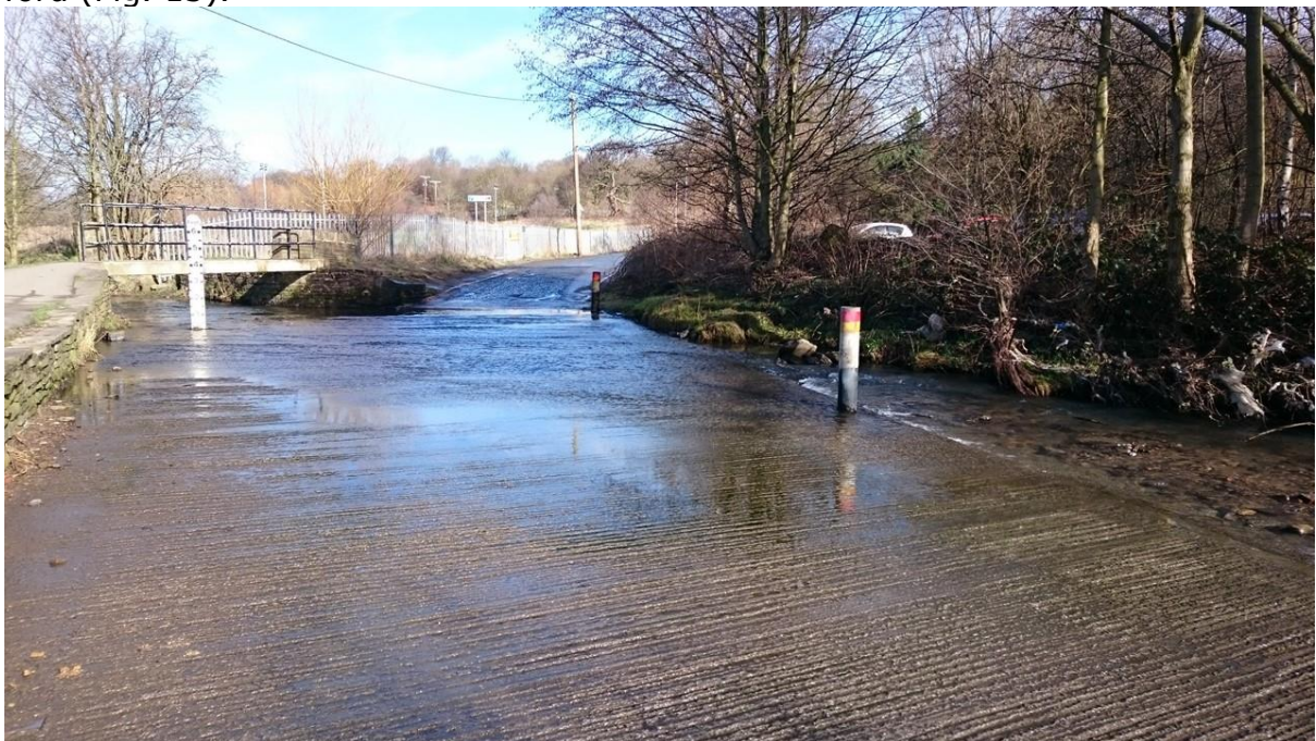
Figure 15: Concrete ford at SE14715 23643 – a serious barrier to fish migration.
