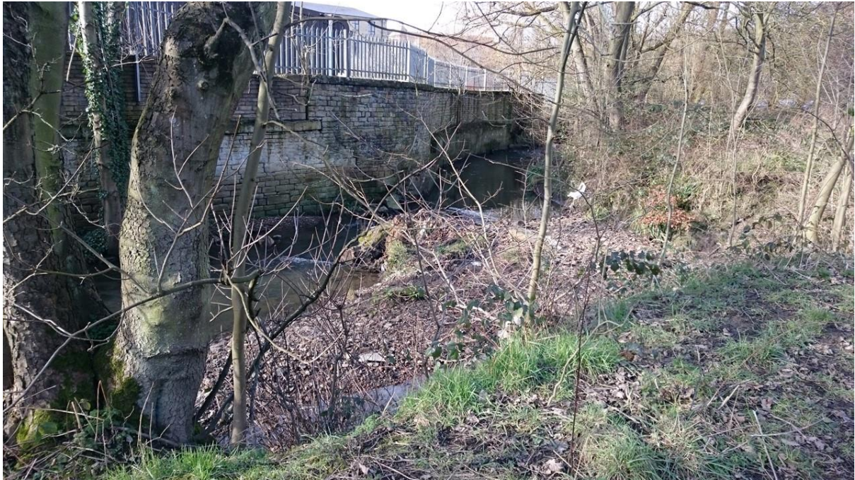
Figure 14: Remains of an old weir and associated gravel-bar depositional feature. At the far bank, the weir structure has washed away so that the original bed level is close to being reinstated. This has restored fish passage and has also delivered habitat improvements upstream and downstream.
