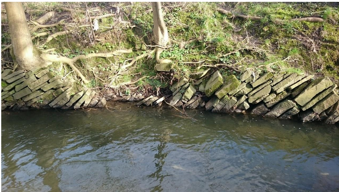
Figure 6: A scour pool of impressive depth formed by a sharp bend on the river. Both the depth and the tight angle of the bend are enabled by the resistance of the banks resulting – not only from the old stonework – but also from the deep root-structure of woody vegetation. Over the longer-term, the self-regenerating living reinforcements (tree roots) will be more reliable than temporary built stonework for ensuring the resistance of banks to lateral erosion.
