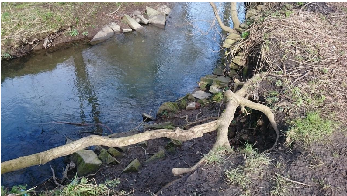
Figure 12: Gradual collapse of stonework (expensive to maintain) may highlight the desirability of establishing woody vegetation that will automatically regulate rates of bank erosion with little requirement for additional intervention or cost.
