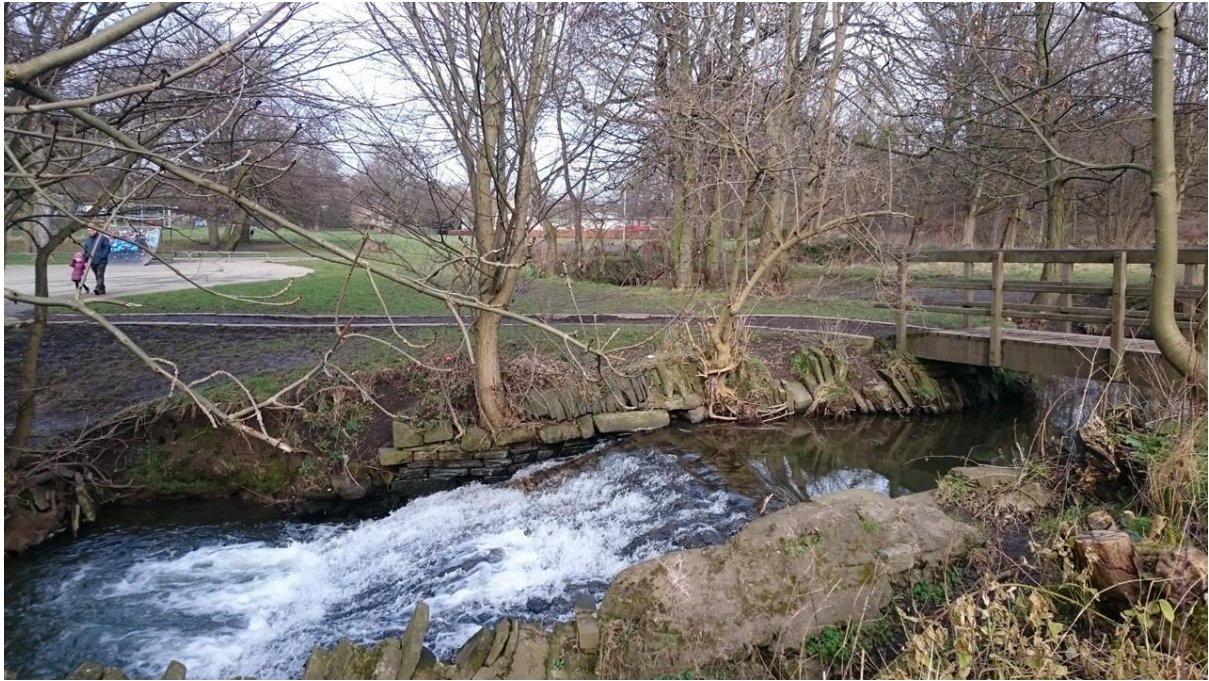
Figure 9: The sloping face of the weir with its shallow, fast flow of water is a complete barrier to upstream migration of trout and other fish. White water indicates the air entrained within the flow that removes the ability of fish to swim.
