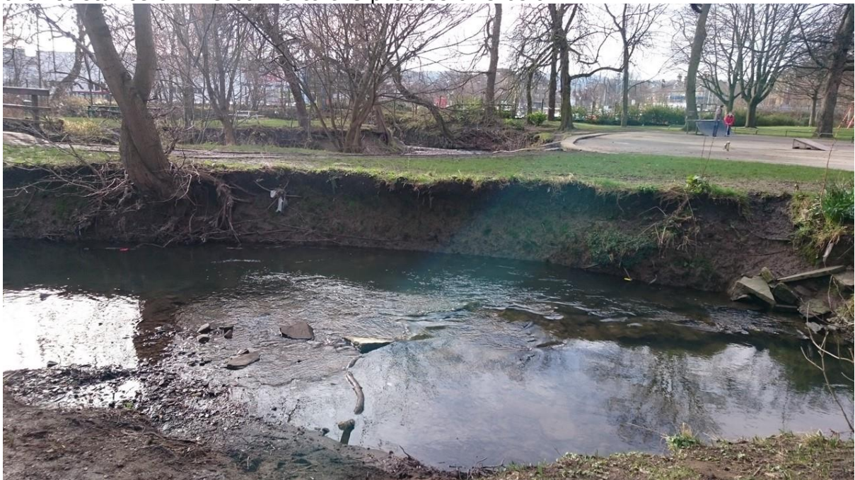
Figure 10: Looking downstream from above the weir, the hand-rail can be seen on the footbridge over the weir top left of frame (also visible in Fig. 9). The shallow root system caused and maintained by mowing of vegetation means that the river is cutting its way around the weir.
