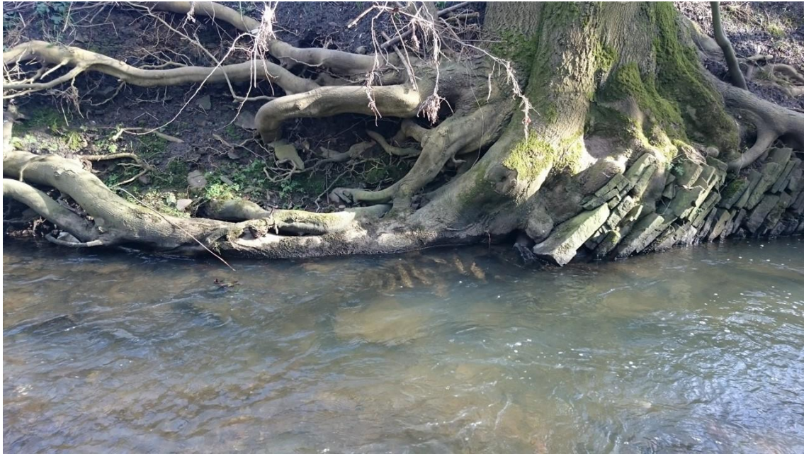
Figure 5: As well as scour-pool creation, the roots of this tree have stabilised and controlled rates of bank erosion after the failure of the stone wall.
