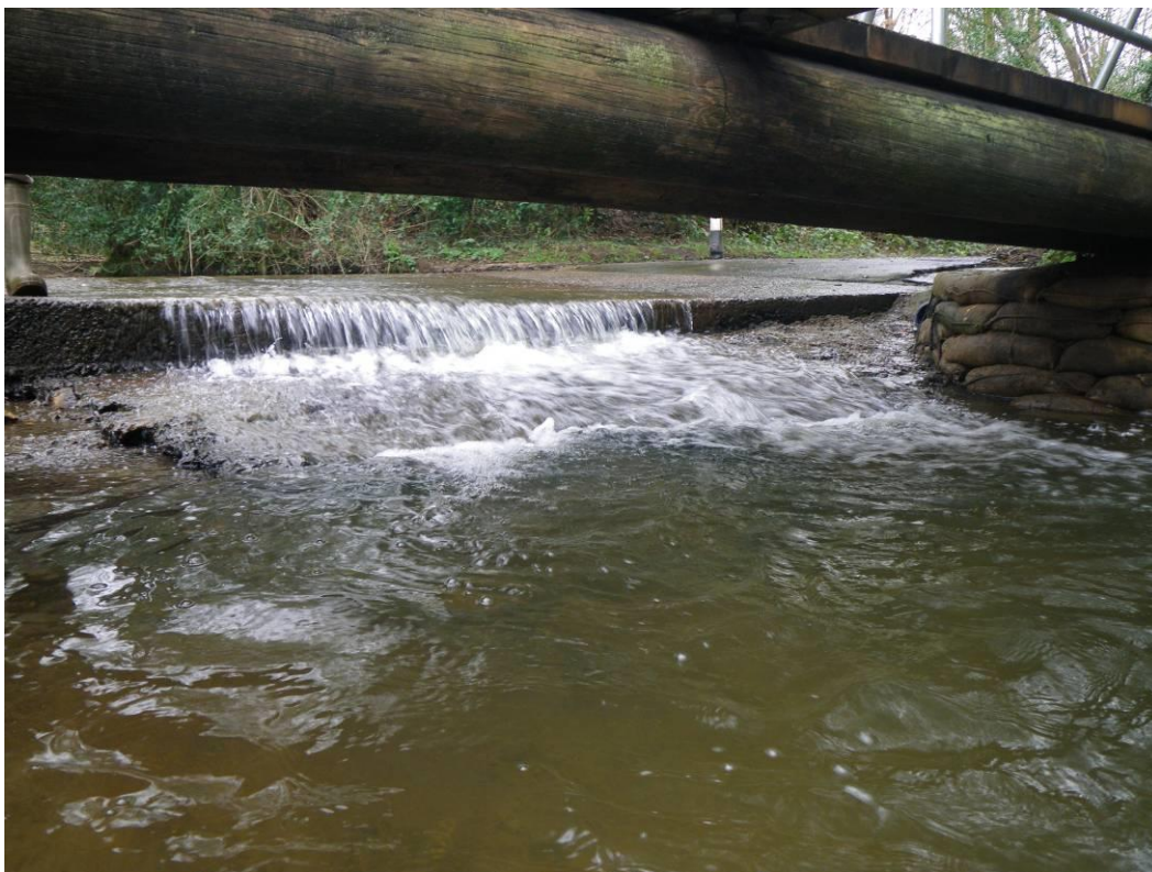
Photo 2. Ford at the top of the stream section. Difficult access for trout.
