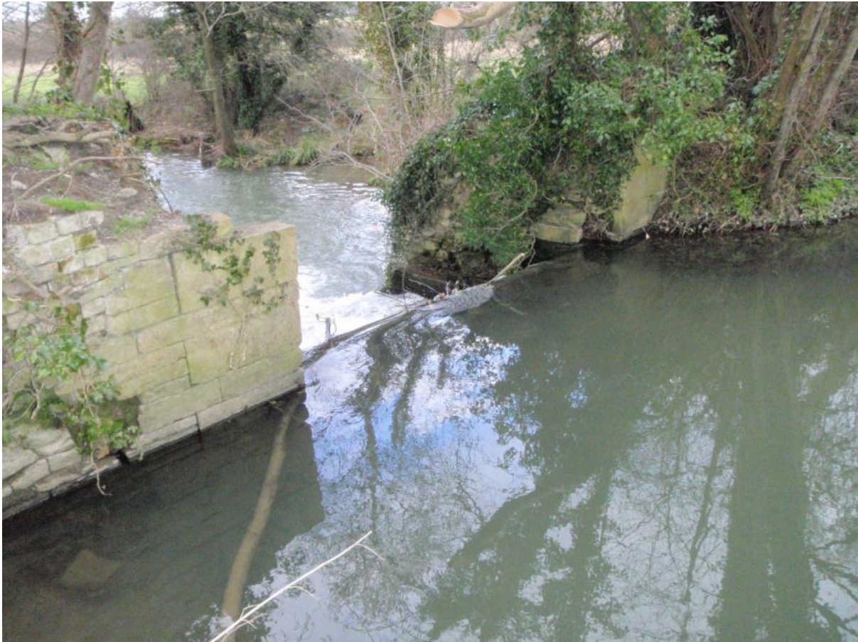
Photo 4: Weir on beat 6 (Ozleworth Brook); note deep slow, sluggish conditions above. The weir's height makes it completely impassable to fish.
