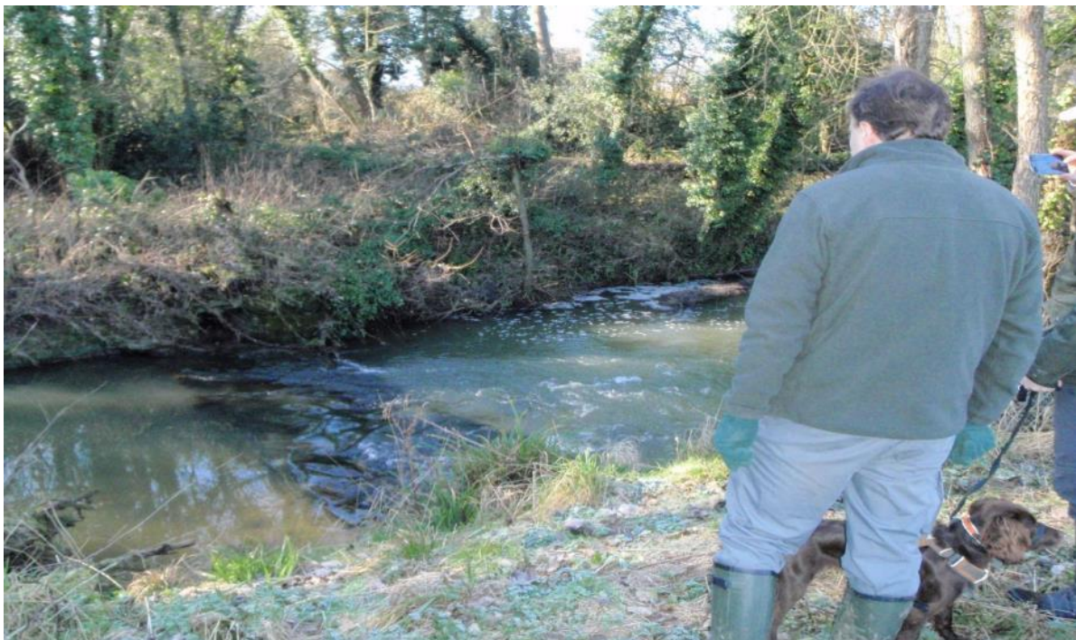
Photo 1: Remains of defunct weir on beat 1; note the base stones are intact allowing fish passage over the top
