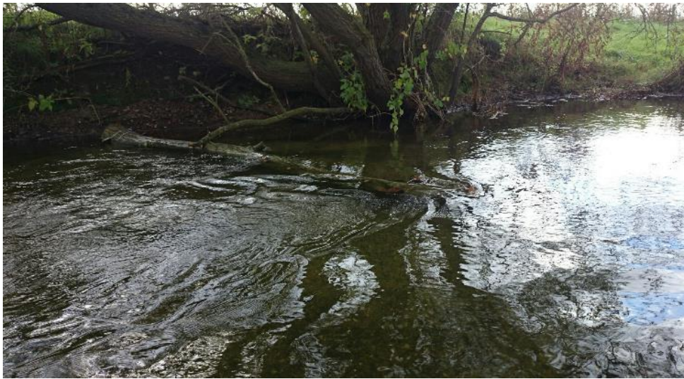
Photo 13: Log deflector pinned with posts and wire (angled upstream, creating bed scour to gravel immediately downstream)
