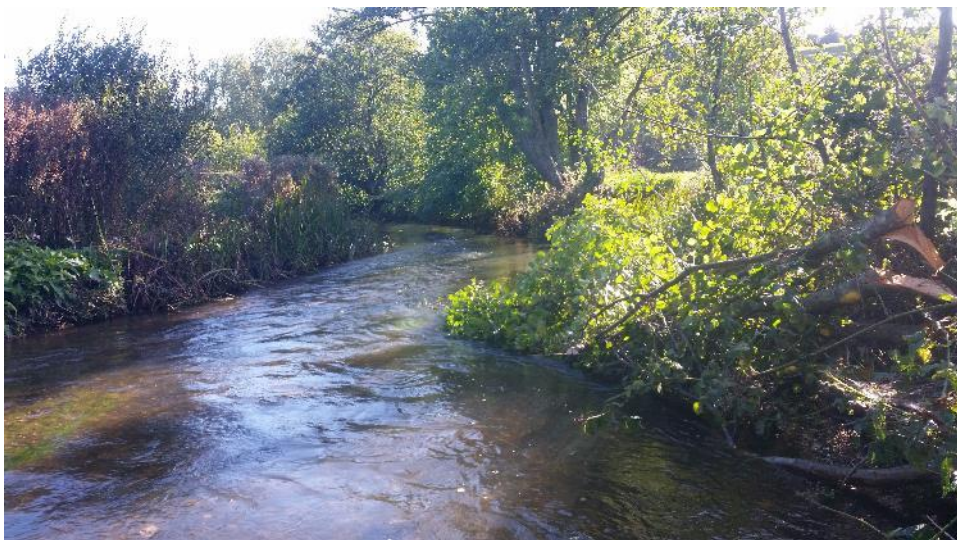
Photo 14: Alder tree with 'living hinge' still attached (angled downstream)
