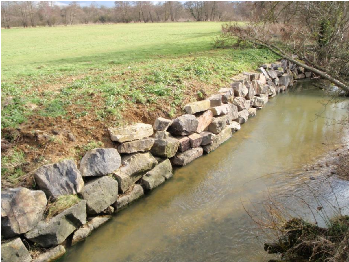
Photo 9: Limestone block repair; the sheer vertical face presents problems for marginal and emergent plants to colonise.
