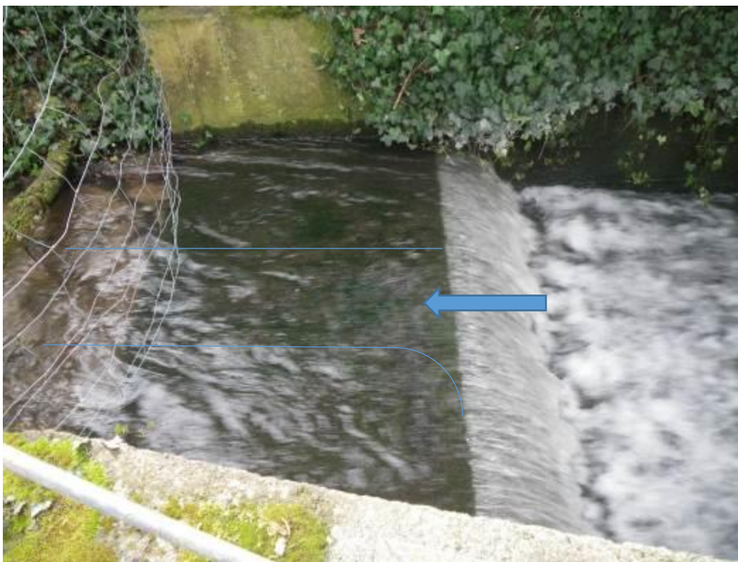
Photo 5. Combination of notch, shaped exit and baulks to create additional depth.
