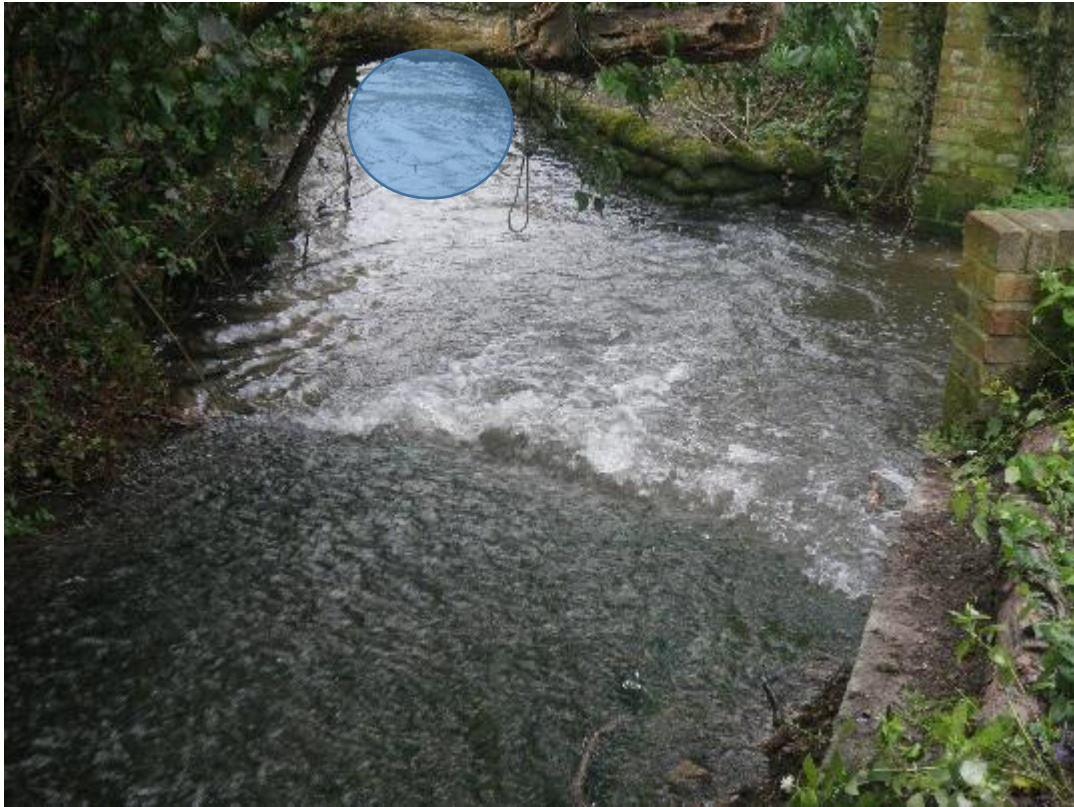
Photo 1. Weir tail. Blue zone indicates approximate location of the stone/gravel pre-barrage.
