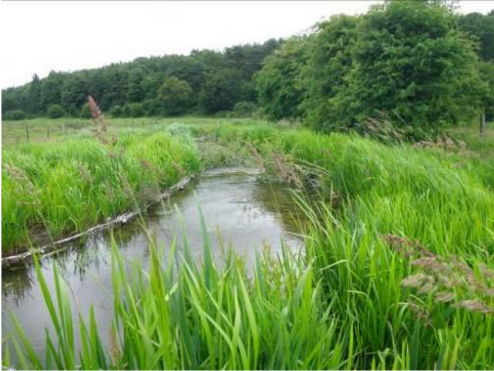
Photo 1. A section of the Candover pinched with hazel faggot revetment, planted with marginal emergent plants and temporarily fenced to promote channel recovery.
