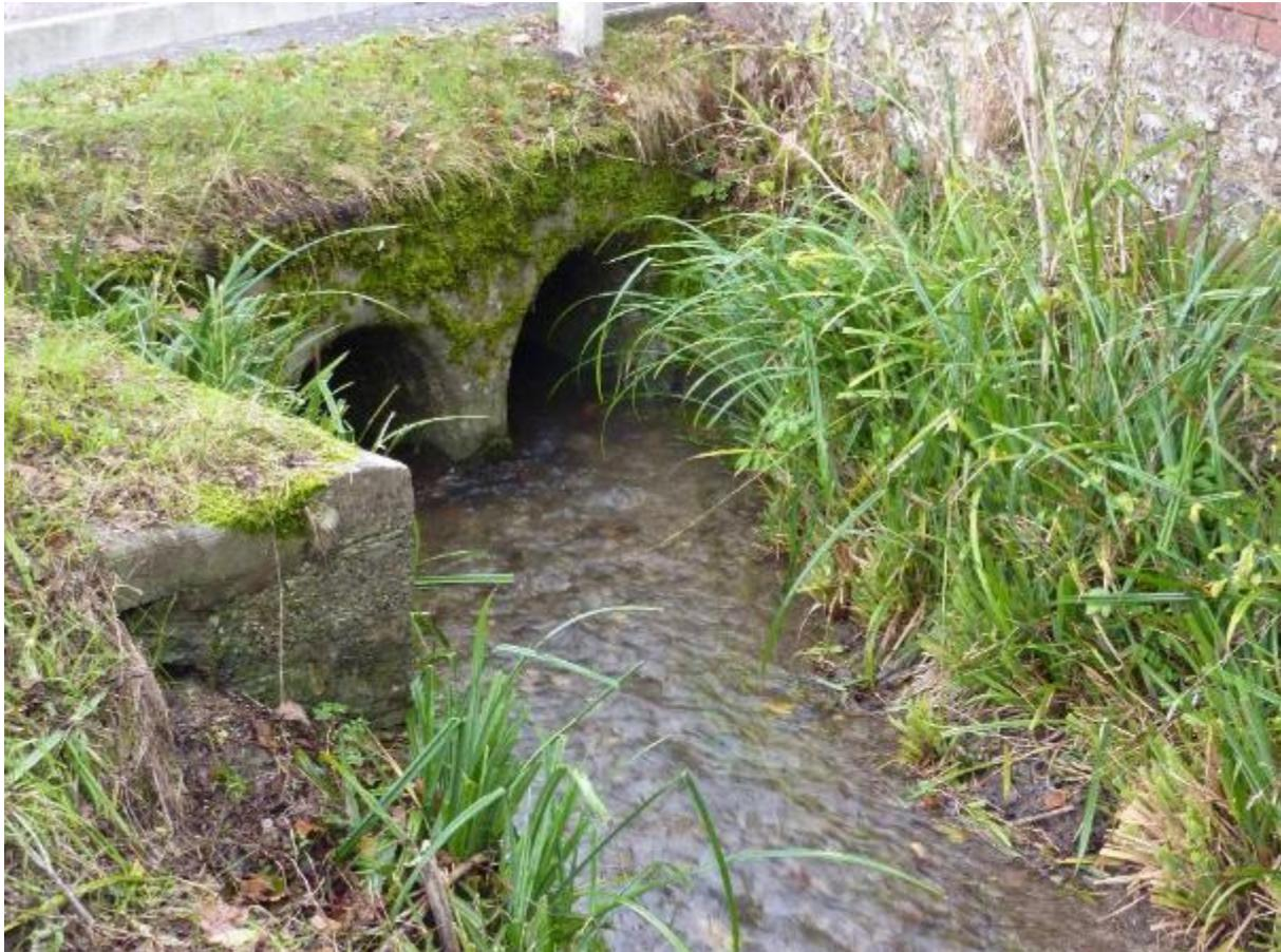
**Figure 5: Double pipe culverts represent an obstacle to fish passage as well as a local flood risk. (However, the soft and natural bank, rich with pendulous sedge, is very beneficial to this stretch of stream)**
