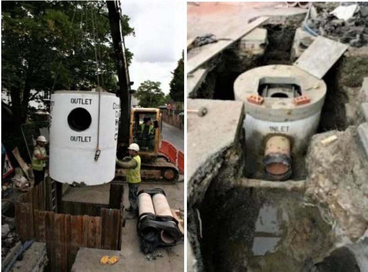
Figure 24: Downstream Defender hydrodynamic vortex chamber silt traps, originally designed for very high volumes of motorway runoff, being installed to intercept sediment in surface water drains near the River Wandle in south London (Photos: SERT)
