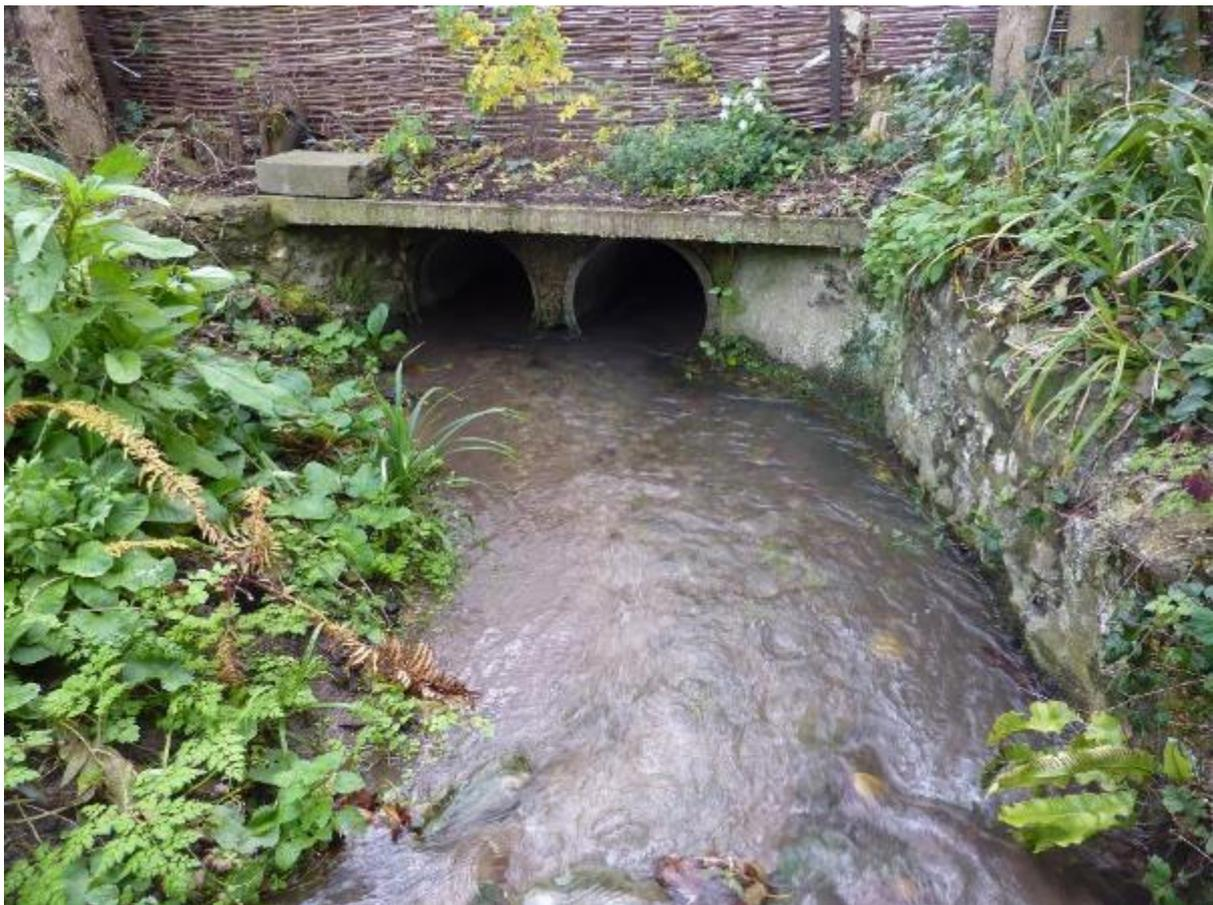
**Figure 14: The upstream end of the culvert under Robins Garden: undersized pipe culverts create flood risk for nearby properties, and could be broken out to make more space for water in this urbanised landscape**
