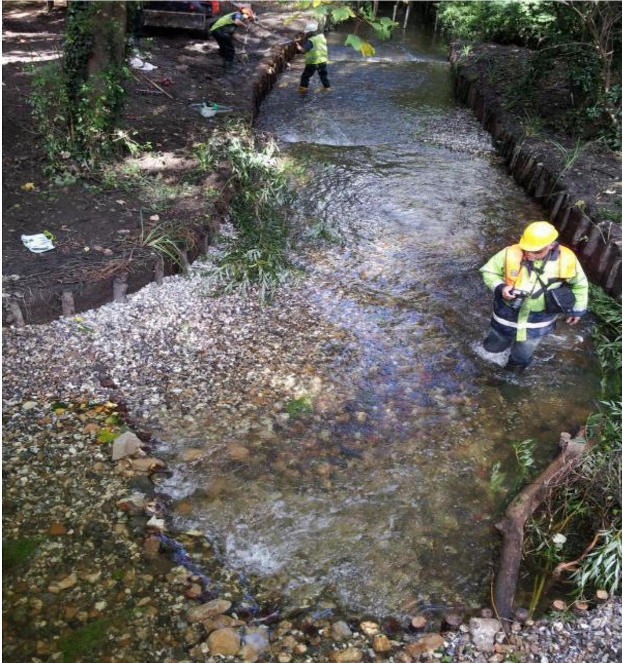
**Figure 29: A nature-like rock ramp, constructed to replace a redundant weir on a small side channel of the River Wandle**
