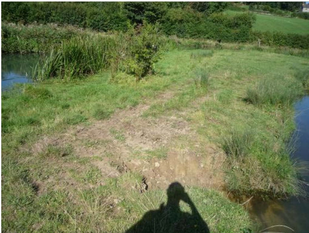
A tight meander with evidence of potentially serious bank erosion due to cattle poaching in the foreground
