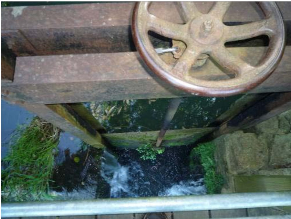
Undershot hatch on the weir screwed down to maintain upstream levels.
