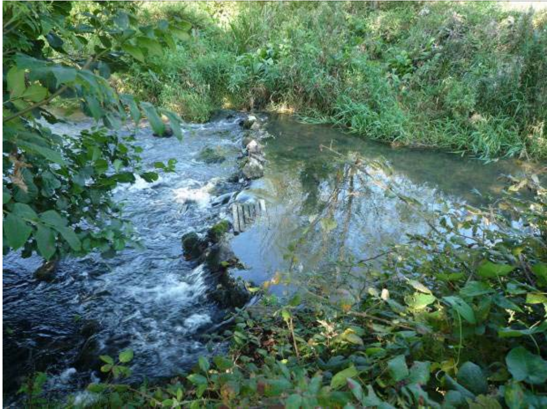
A Low stone weir reducing upstream water velocities. Notching the centre third will help to improve habitat for wild trout in the section upstream
