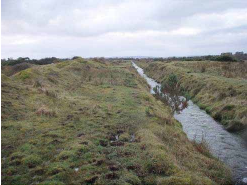
Photo 13 Ballynulty Stream – straightened and dredged (spoil heaps on LHB); the subject of a habitat improvement project
