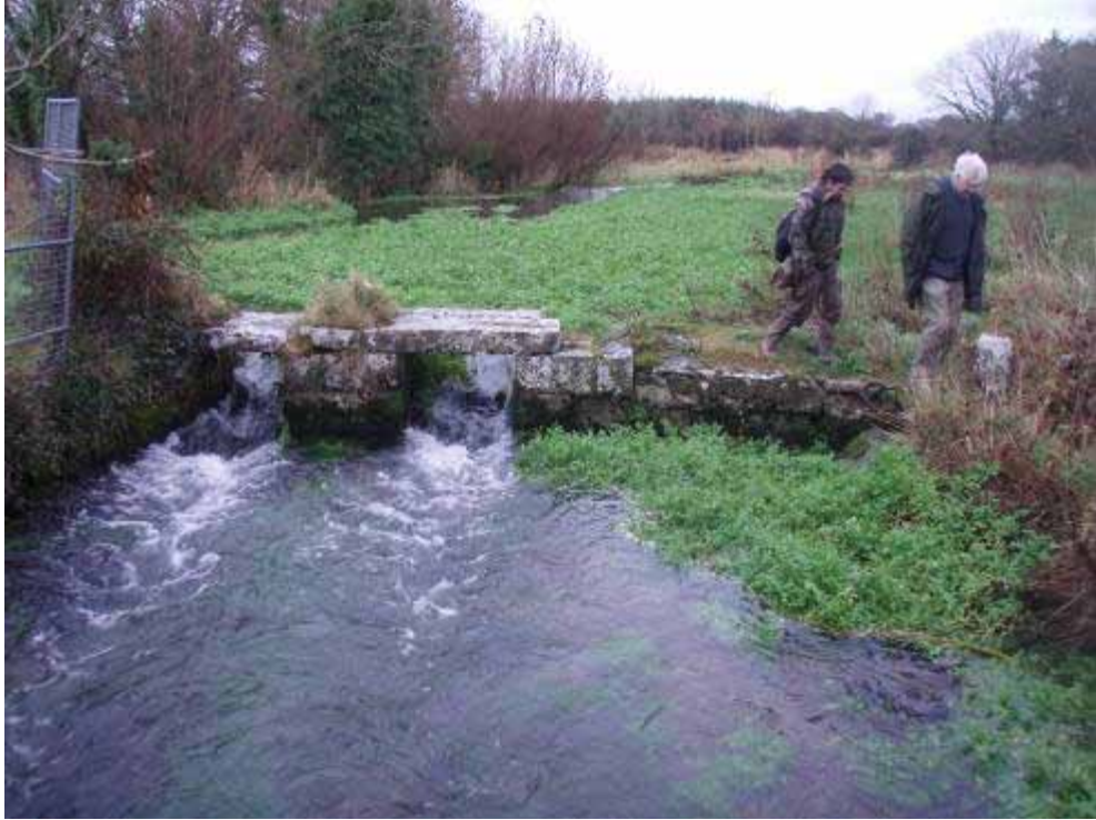
Photo 1 Former mill pond, now with open sluices. During the operation of the mill, boards would have been placed in the sluices, and the overspill is where the people are walking. The mill is to the left of the picture.
