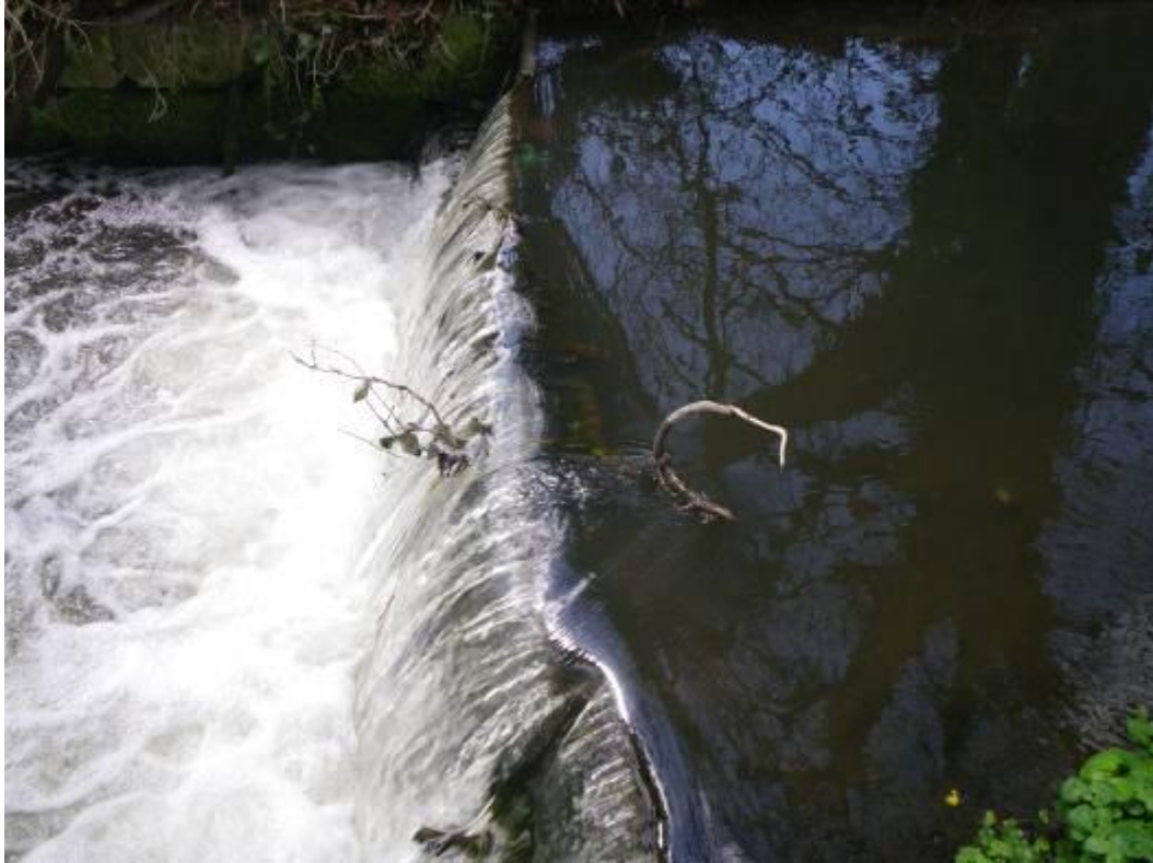
Photo 7. Weir crest could be removed, modified or bypassed.
