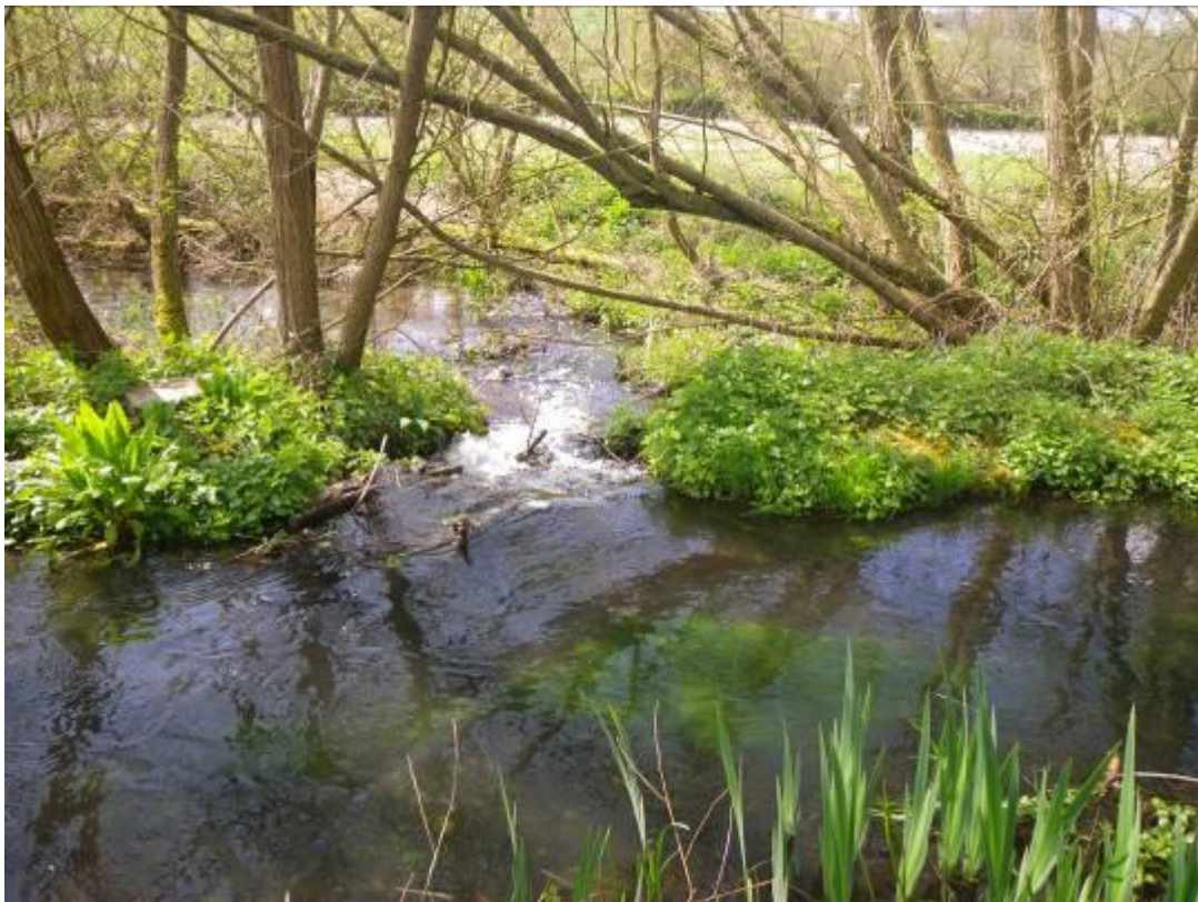
Photo 9. Bank breach above the weir. There is no "do-nothing" option here.
