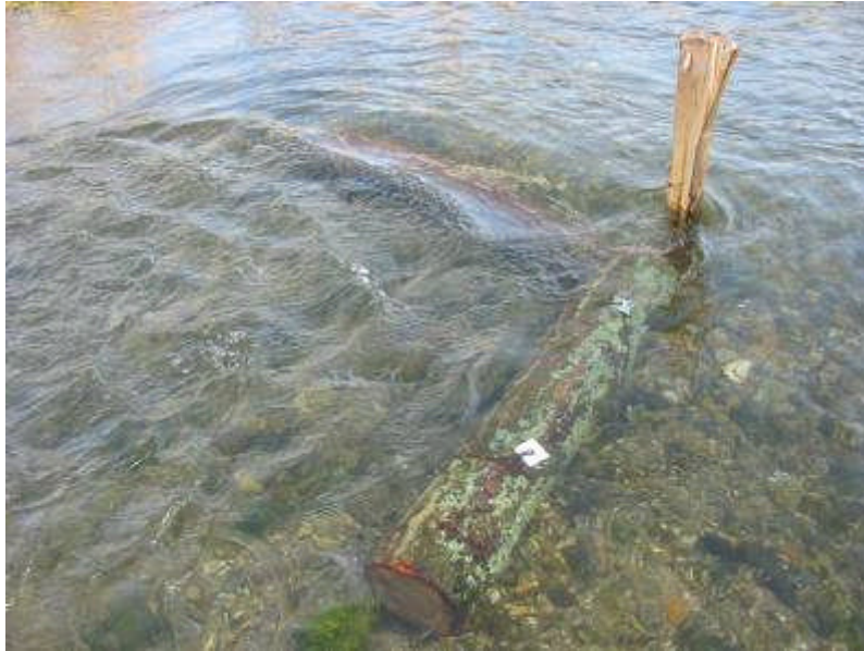
Paired LWD limbs used to create a 'v' shaped deflector. Note rebar and steel washer fixing
