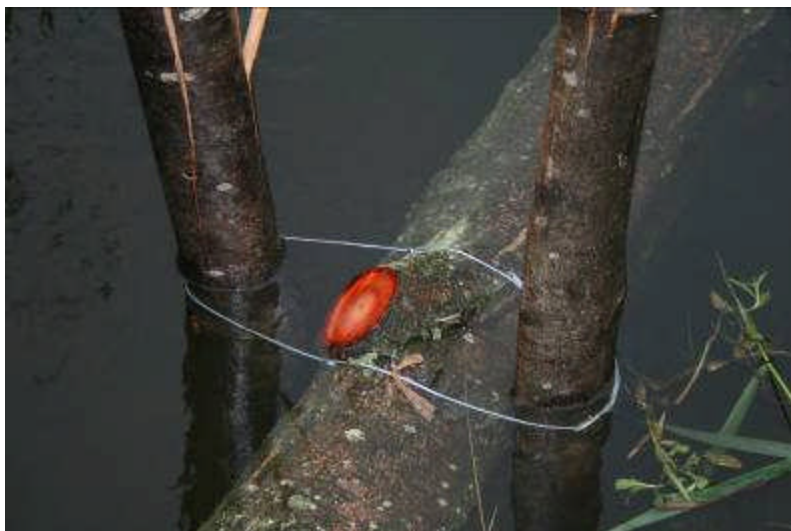
.... And additional fixing using stakes and wire
