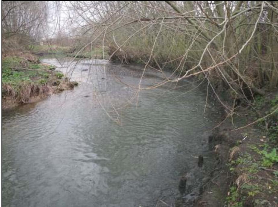
Figure 10. The enhanced river channel at Tokyngton Park that previously ran through a concrete channel.
