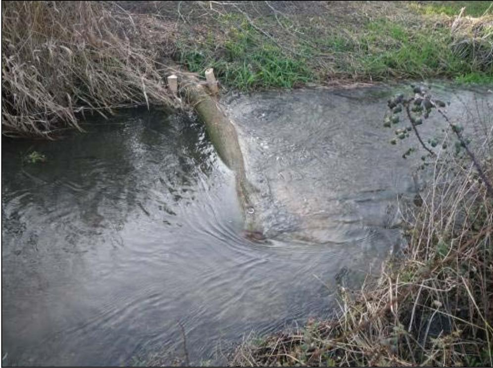
Figure 12. An example of a LWD flow deflector secured to the river bed and designed to erode and redistribute river bed gravels.
