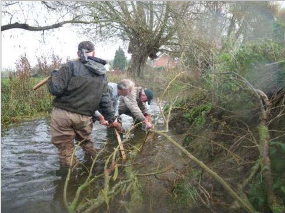
Figure 13. CWD being laid up against the margin on the River Wey in Surrey.
