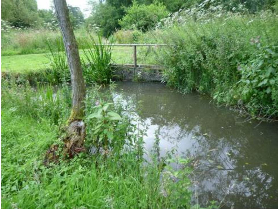
Photo 3 Water off-take feeding into the hatchery ponds, which relies on the water level maintained by the weir downstream of this picture (NGR SK2433143031).
