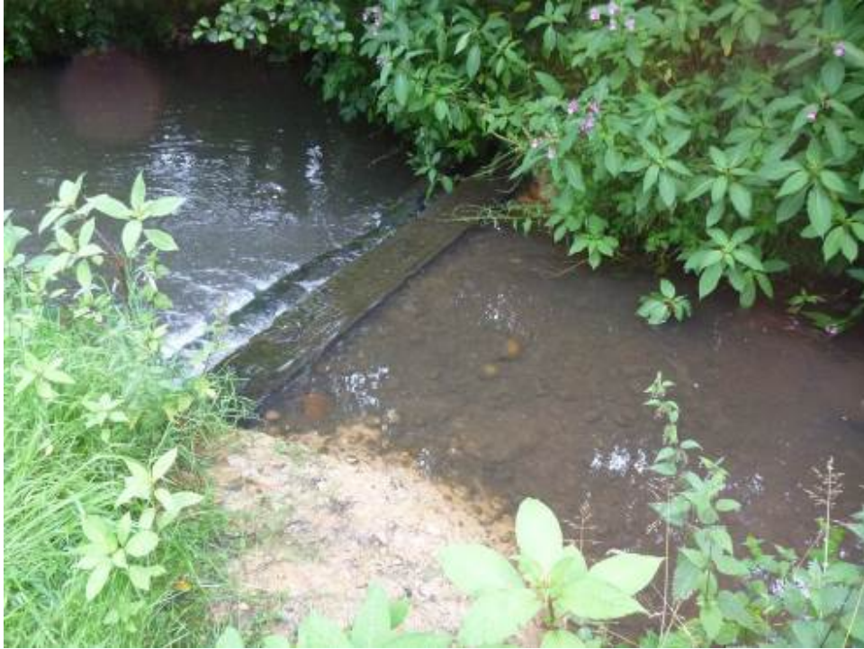
Photo 1 Accumulation of gravel upstream of a weir, trapping suitably-sized trout spawning medium in an unsuitable area for spawning. Also note the accumulation of silt amongst the gravel.
