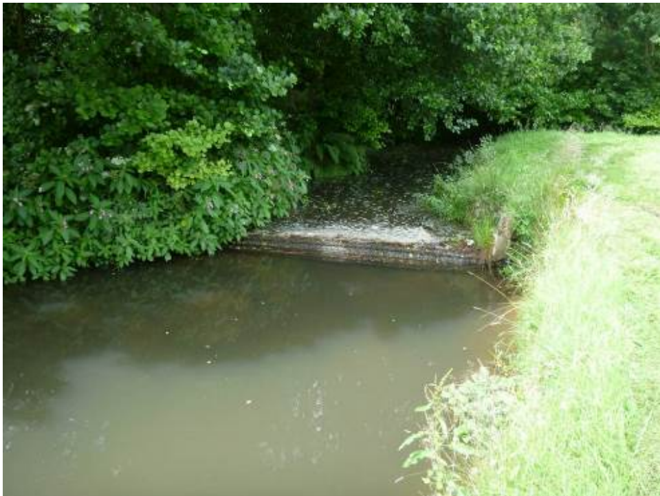
Photo 11 No flow over the weir near the Bradley Brook confluence – further investigation is required to clarify the flow pathway here.
