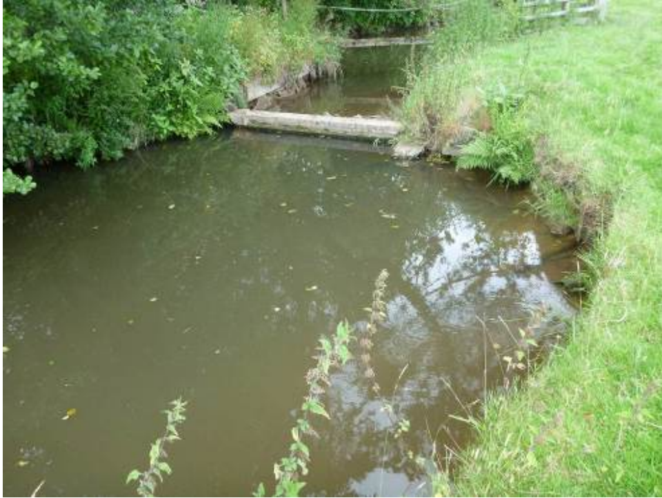
Photo 10 Plastic drainage pipes discharge water to the brook from the true left bank (right of picture) – the outflow from Sandy's Lake? Note the lack of flow over the weir upstream, resulting from the diversion of flow through the hatchery ponds which lie on the true right bank adjacent to this area.
