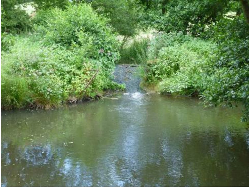
Photo 7 Weir downstream of the footbridge below Dam Farm (NGR SK2436142611) which maintains water levels for the mill leat to Brailsford Mill (requires further investigation).
