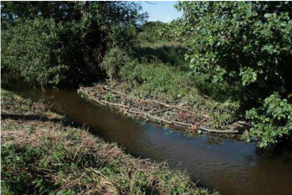
Photo 19 Example of a brushwood mattress
