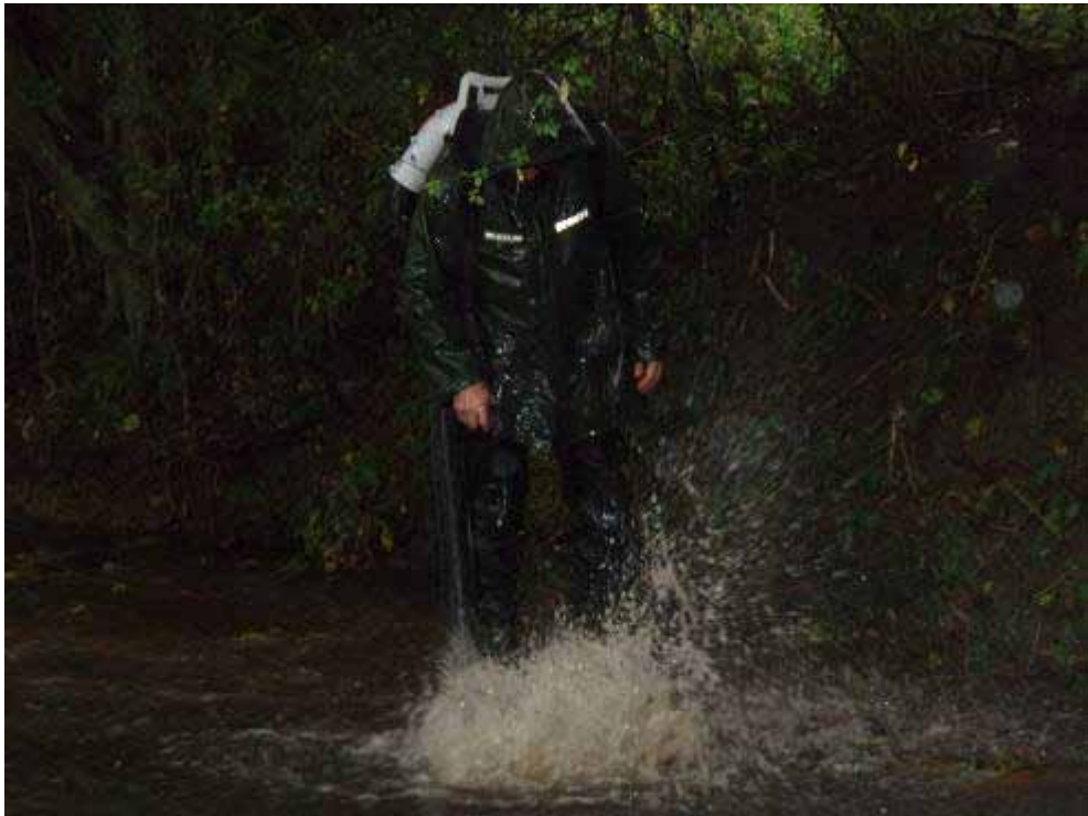
Photo 21 Gravel cleaning with a portable leaf blower
