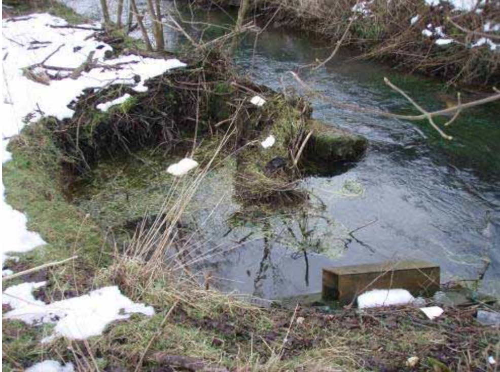
Photo 20 Area suitable for backfilling with brushwood
