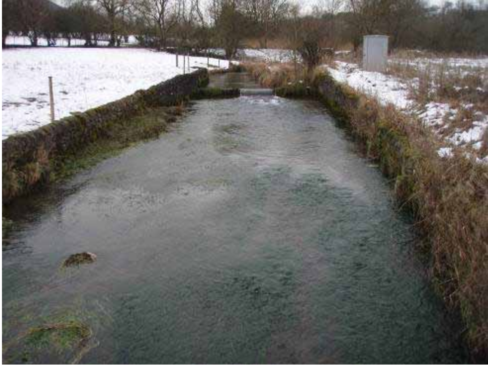
Photo 9 Gauging weir and walled, wide, shallow channel
