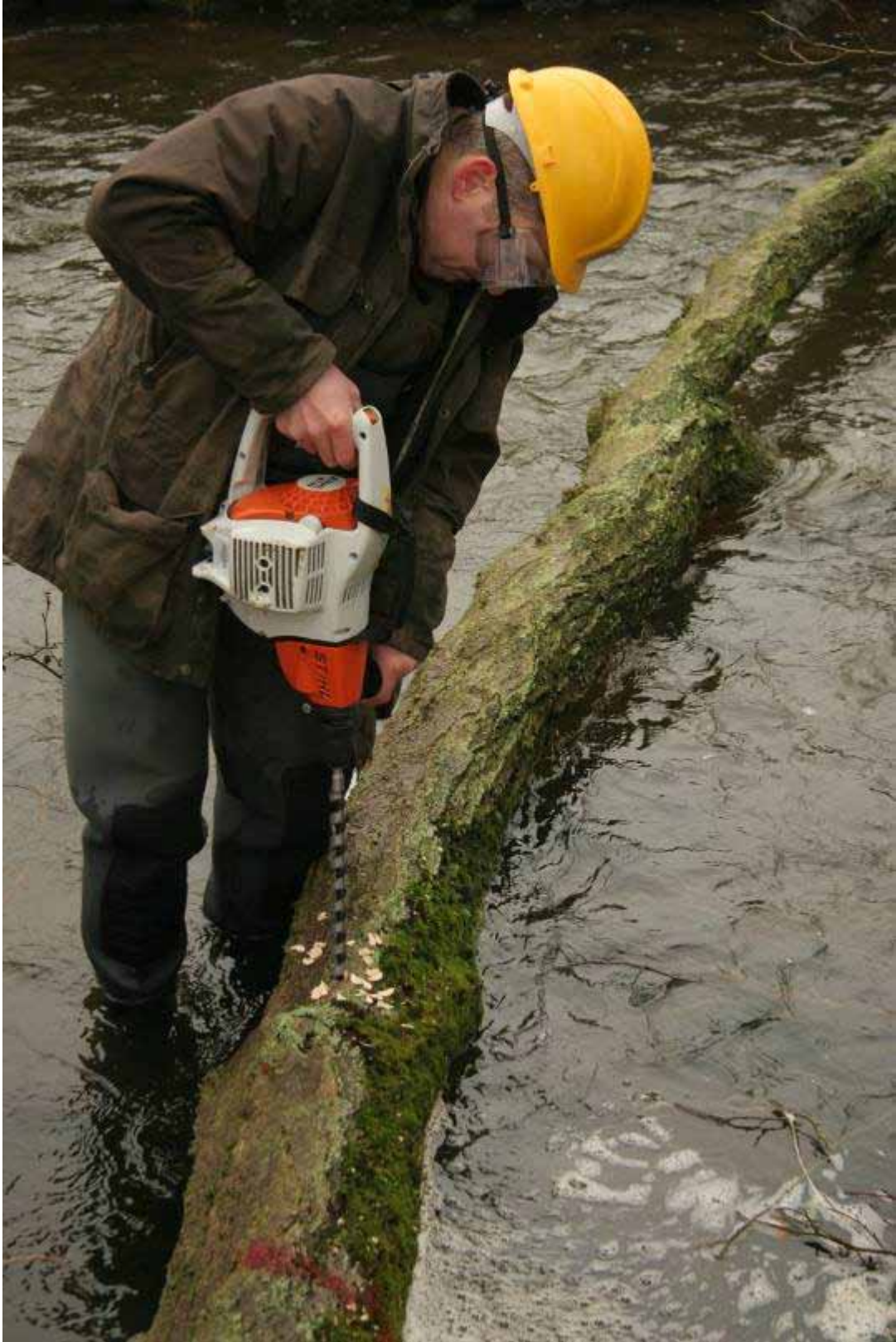
Photo 17 Installing LWD
