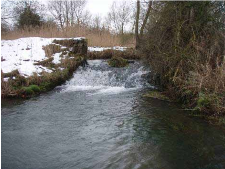
Photo 7 Weir alongside old pond
