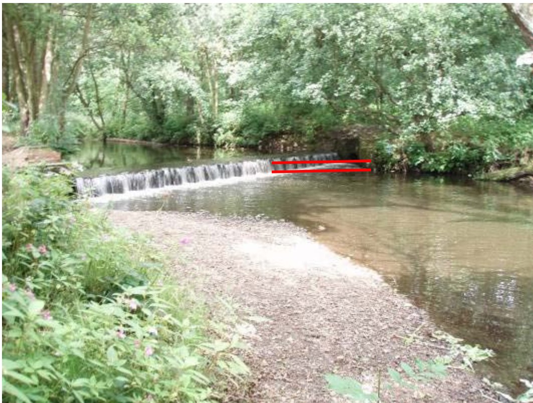
Photo 6 Pipe weir with potential location of pre-barrage
