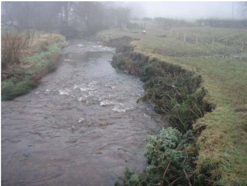
Photo 3 Soft revetment techniques can successfully reduce erosion rates and consolidate banks (River Manifold, Staffordshire)
