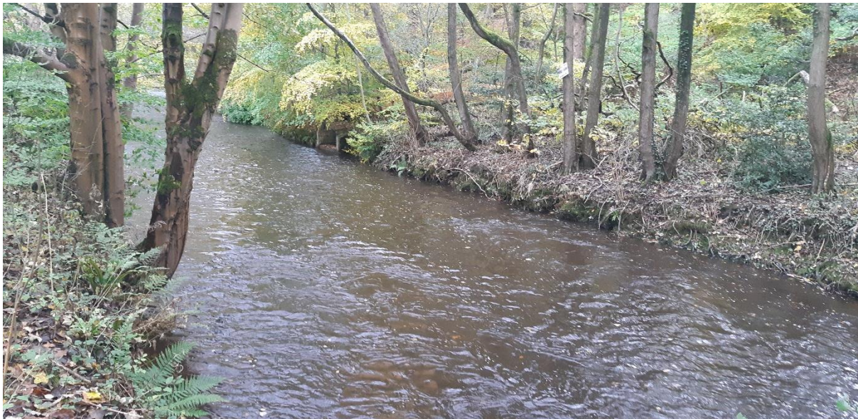
Figure 5: This section appears to have been straightened in the past. Rock revetments are often stabilised by the roots from a line of riparian trees, as is the case here. However, this does create opportunities for stable, cross-channel large woody material features similar to the naturally arising example shown in Fig.3
