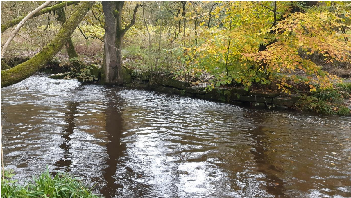
Figure 17: Low blockstone revetment visible on the opposite bank. This will eventually erode away and the growth of bankside trees indicates nature is in the process of colonising these remaining structures.
