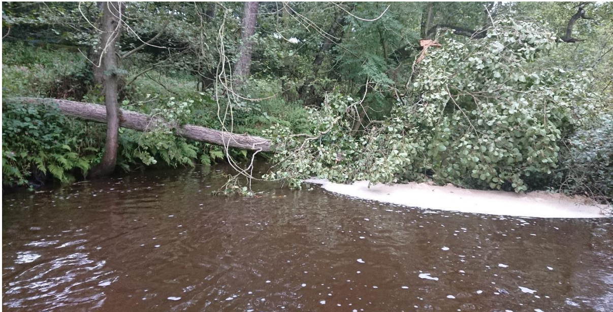
Figure 21: Wedged cross-channel tree habitat feature installed on the River Washburn – note the length and mass of main trunk remaining on the bank, lodged between standing, live trees (left of frame) as well as the space beneath the main trunk to allow flow to pass through for much of the full channel width.
