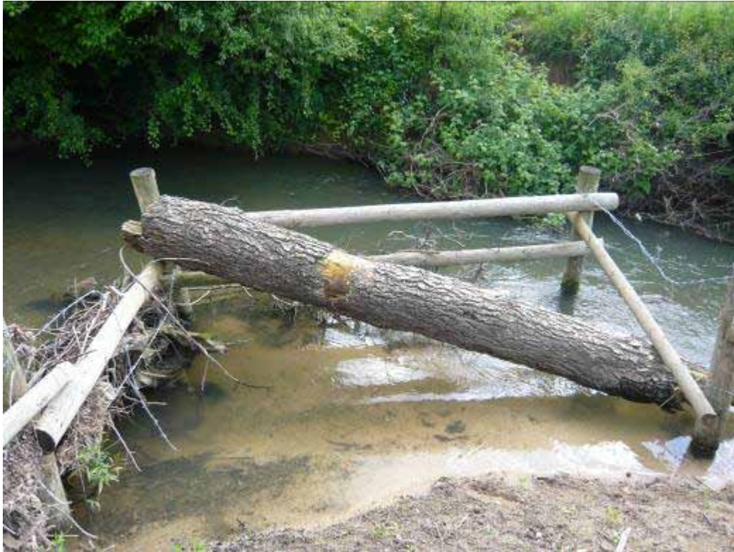
The Box brook has the power to mobilise large trees so it is vital to secure LWD when using it to promote trout habitat
