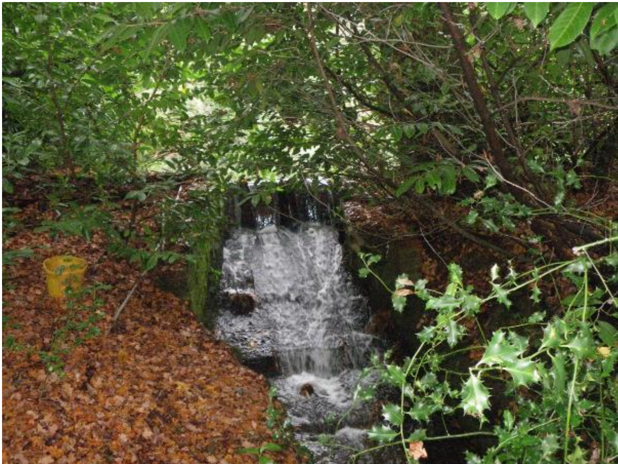
Photo 1. The outfall sluice and dam
