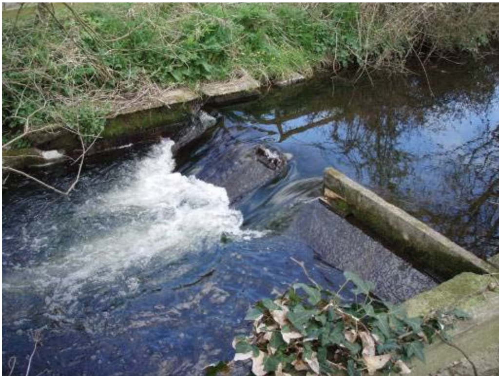
Photo 4 Outflow from Llyn Coron into the Afon Ffraw. The weir and boards were intended to raise lake water levels in an attempt to combat algae blooms.
