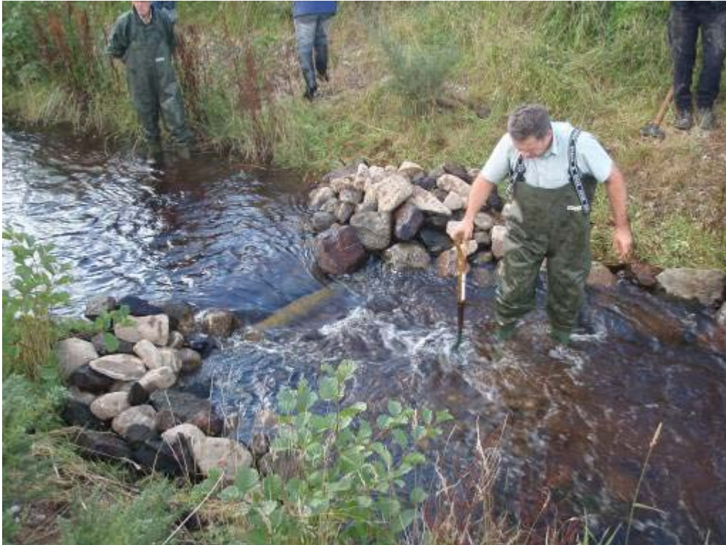
Photo 25 Example of a pinch point created using logs and stone to encourage bed scour and sorting of gravel. On the smaller watercourses on the Bodorgan Estate, large boulders could quickly and easily be positioned with an excavator to create the same effect.
