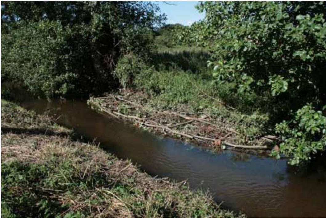
Photo 15 Example of brushwood mattress installed in the River Glaven, Norfolk
