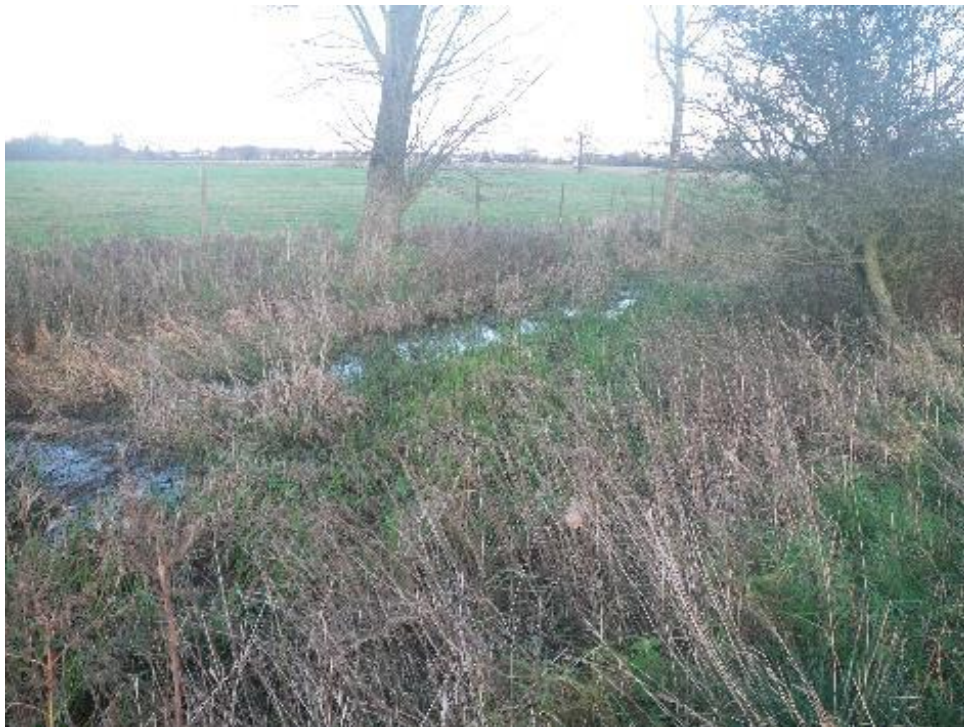
Photo 2. The downstream "dog-leg" channel which picks up flow from various ditch systems and is connected to the main river at its downstream end.
