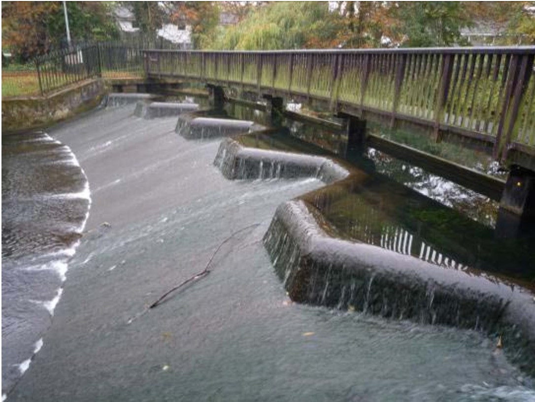
The huge fixed crest labyrinth weir downstream of the bottom boundary.
