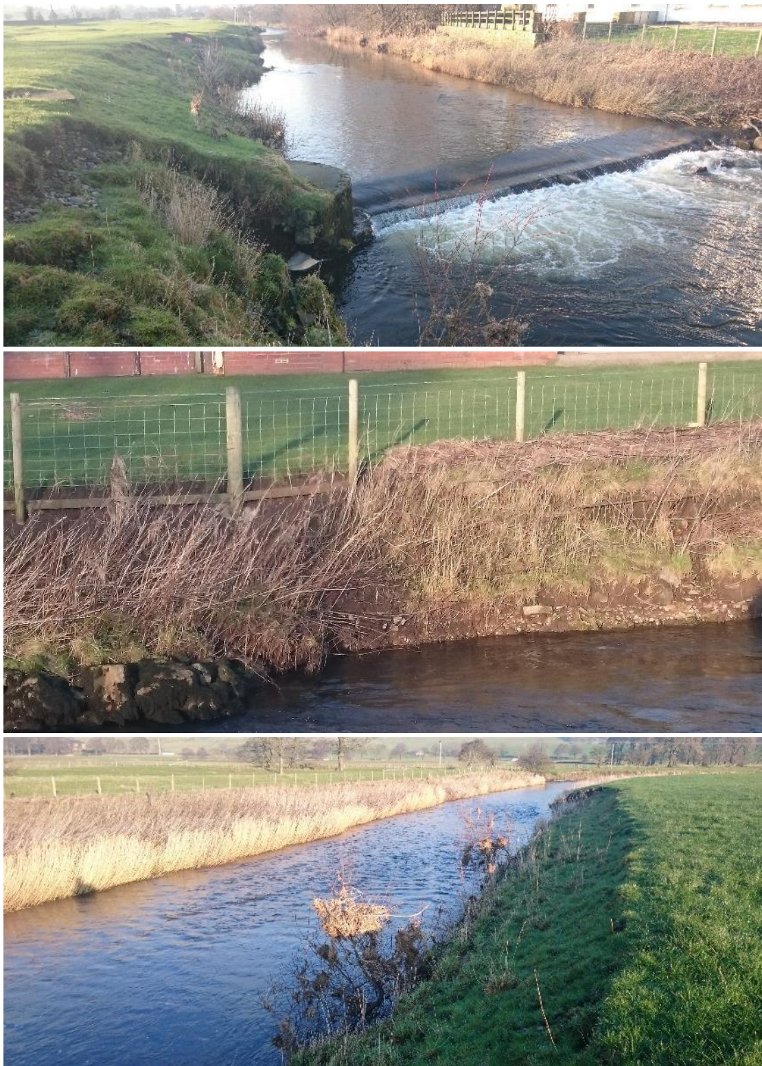
Fig 5. Upper panel: pipe and concrete / stone structures causing impounding u/s. Mid panel: the fence-line becoming vulnerable to erosion, even on the ungrazed LB because of the eddy erosion from the weir structures and insufficient vegetative buffer zone; behind the fence, the lawn is mown. Lower panel: looking d/s at the straightened channel which is essentially one long glide with little riparian cover; two goat willows have managed to establish out of reach of livestock grazing.
