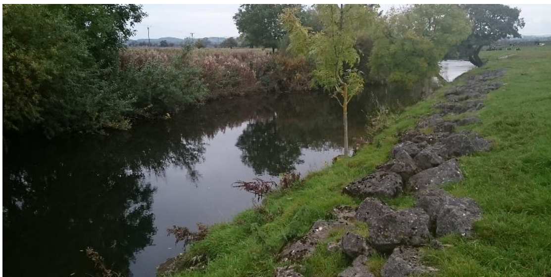
Fig 14. Rock armoring is apparent in many locations, including some straightened sections like this, presumably to prevent the river cutting toward the enormous flood relief bund that has been built on the LB.
