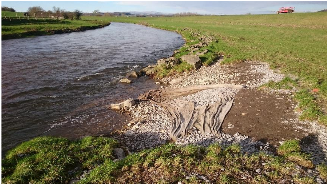
Fig 18. A formalised cattle drink at the d/s end of the glide in Fig 17 has been severely damaged in the recent winter spates. Note the ~3-4m bunding allegedly for flood water storage on the LB (trailer parked on the top).
