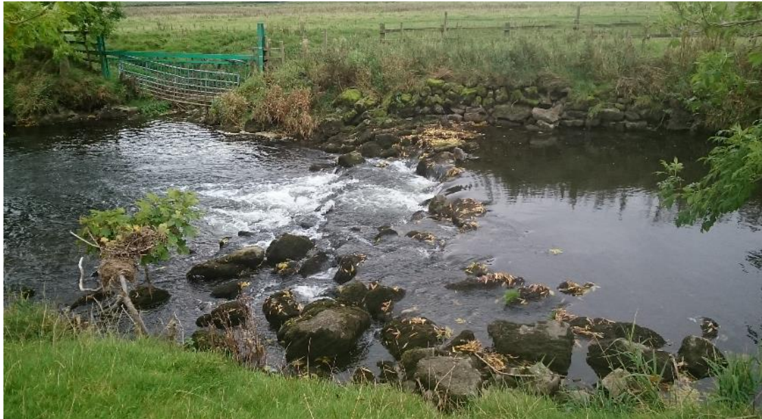
Fig 16. The uppermost weir introduced by the Club. All are in a poor state of repair and even under relatively low flow conditions (here in October) this should be easily passable by fish of most sizes and in both directions (but with delay & possible predation issues), due to the plethora of water channels and flow between the rocks. Note the confluence of a small tributary on the RB beneath the debris gate.
