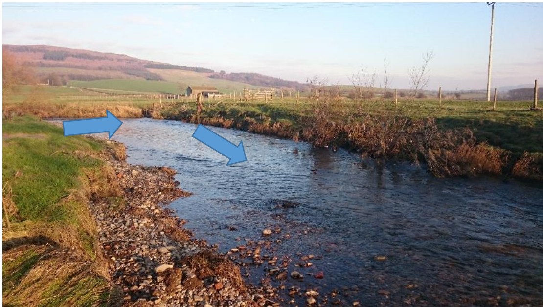
Fig 10. A notable diversion of the flow by rock armouring of the LB to force the river to the right. The LB is protected by livestock exclusion fencing here although it requires maintenance. Aside from the scrubby goat willow, this potential holding pool is very exposed.
