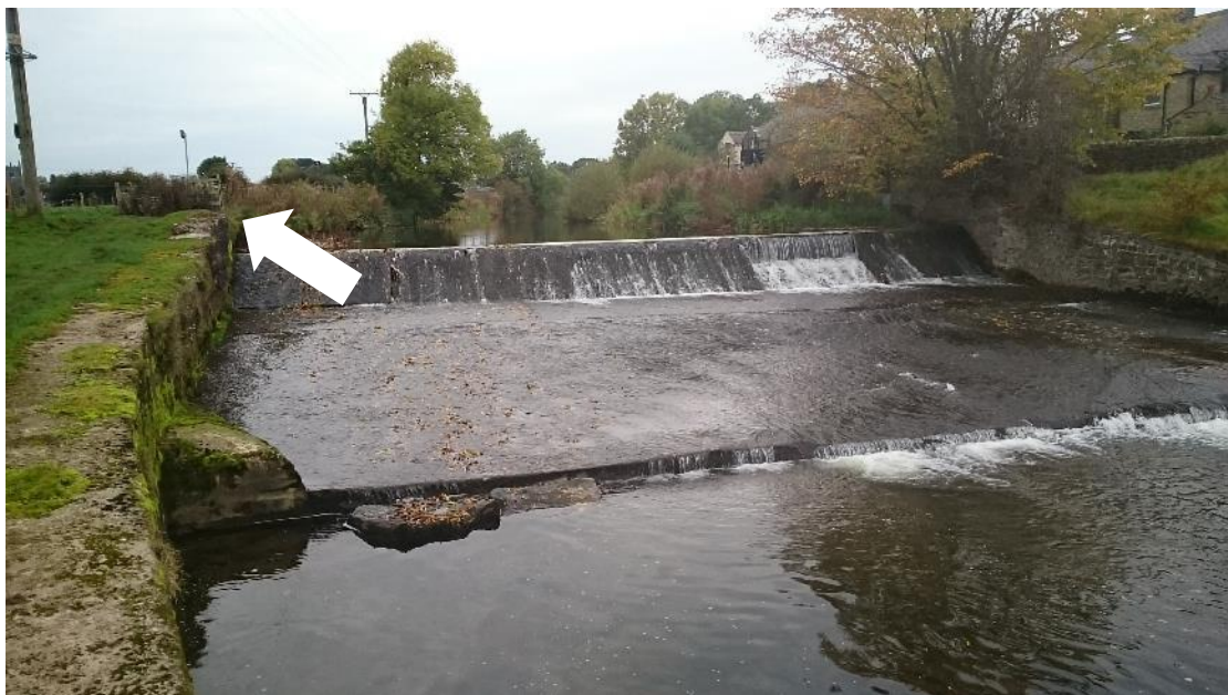
Fig 1. The weir marking the u/s fishing limit of BCAA waters at Gargrave. Major fish passage issues arising from the head-loss ( \sim 3\text{m} ) and perched apron ( >10\text{m} length). Note riparian vegetation protected by fencing immediately u/s on the RB (white arrow).
