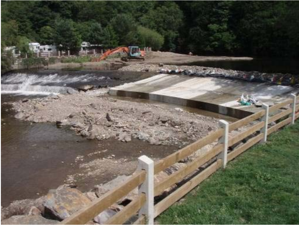
Photo 7 Weir repairs at the camp site
