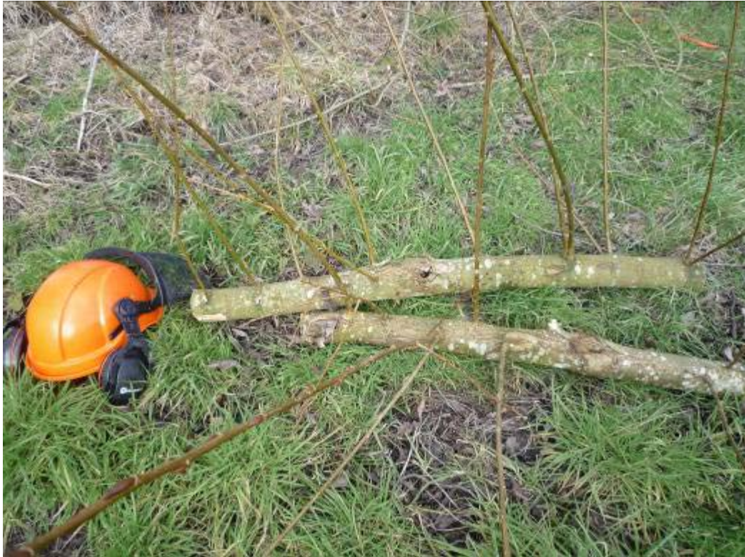
A section of live willow which can be pegged and wired down onto the wet toe of a slumped margin. The willow will set root and protect the face of the eroded bank.
