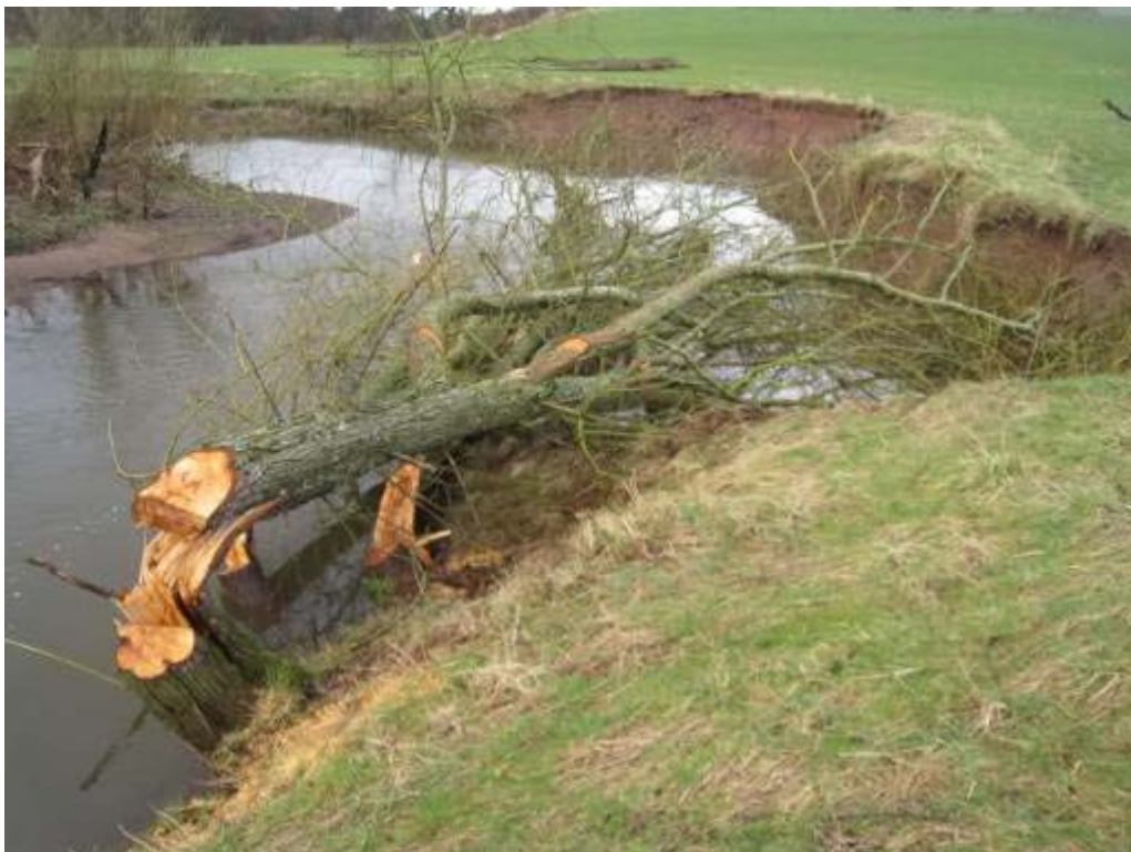
A section of live willow which can be pegged and wired down onto the wet toe of a slumped margin. The willow will set root and protect the face of the eroded bank.
