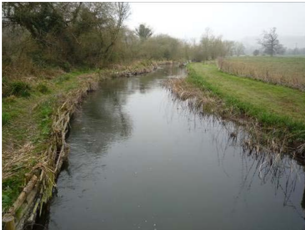
Low banks, deep margins and bank repairs on the outside of a gentle bend
