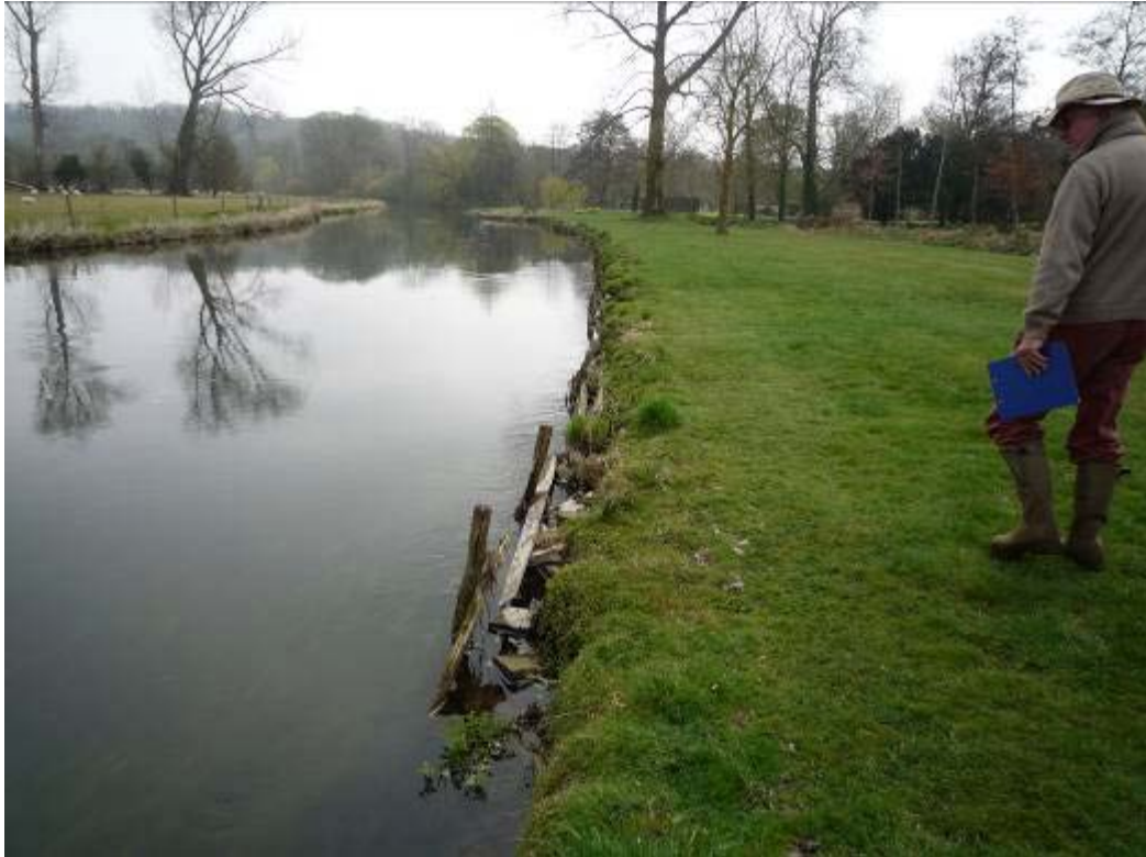
Area adjacent to the formal gardens where attempts to protect the bank have largely failed.
