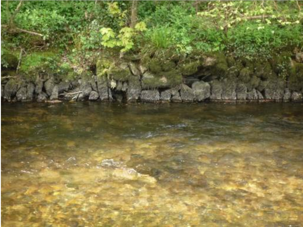
Large stones used to protect the RB from excessive erosion. Some low scrubby cover provided by a small goat willow would soften its appearance and enhance its fish holding capability
