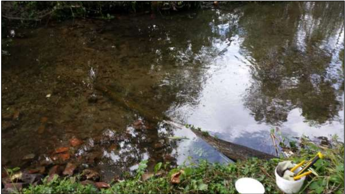
Figure 4: An example of a log deflector facing upstream and keyed in and sloping down from the bank towards the bed.
