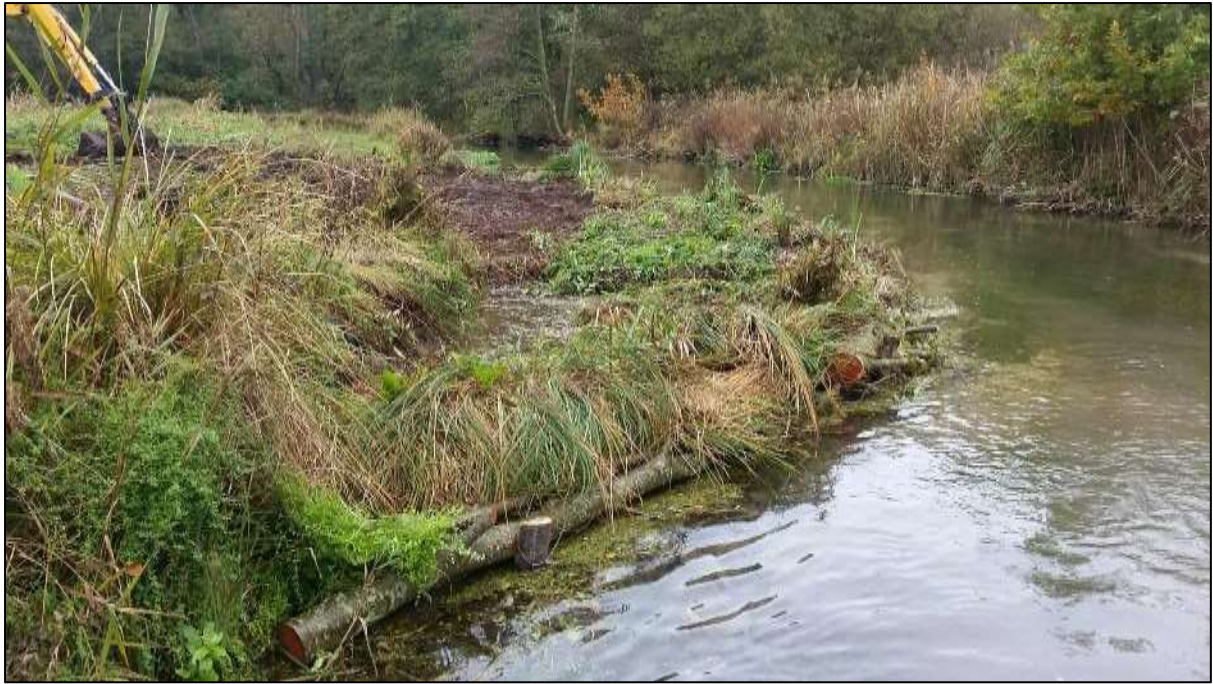
Figure 9: The same site with the bank re-graded to narrow the river, create additional marginal habitat and improve angler access.
