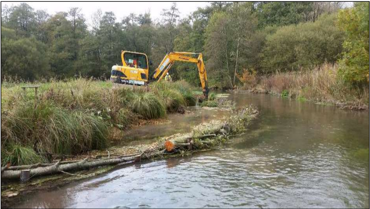
Figure 8: A new bank edge is constructed from site-won woody material on the River Dever, Hampshire.
