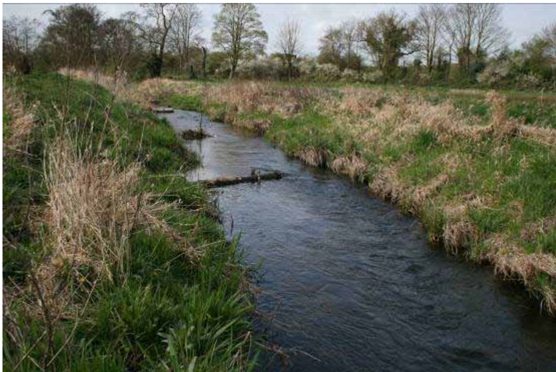
Introduction of LWD at three locations on the Glaven in North Norfolk. (Re-energised flows)
