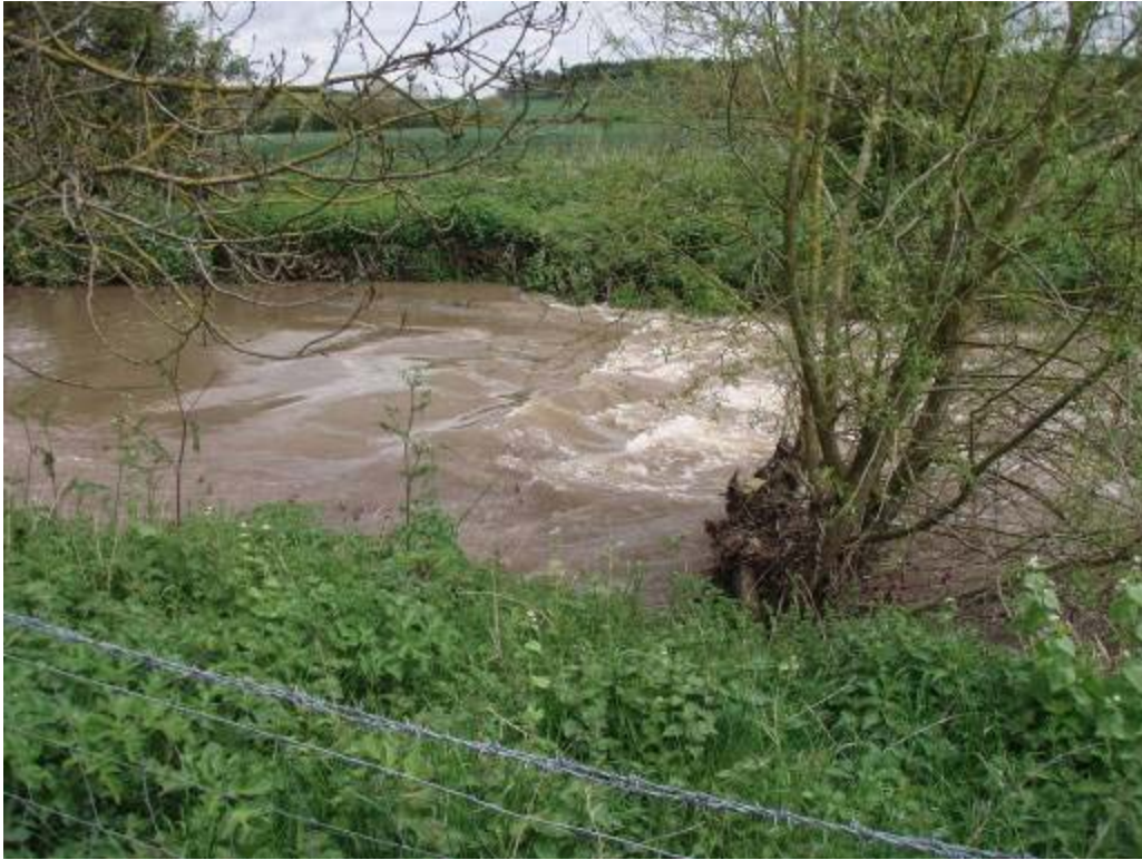
Photo 7 Site 2 – sheet pile weir
