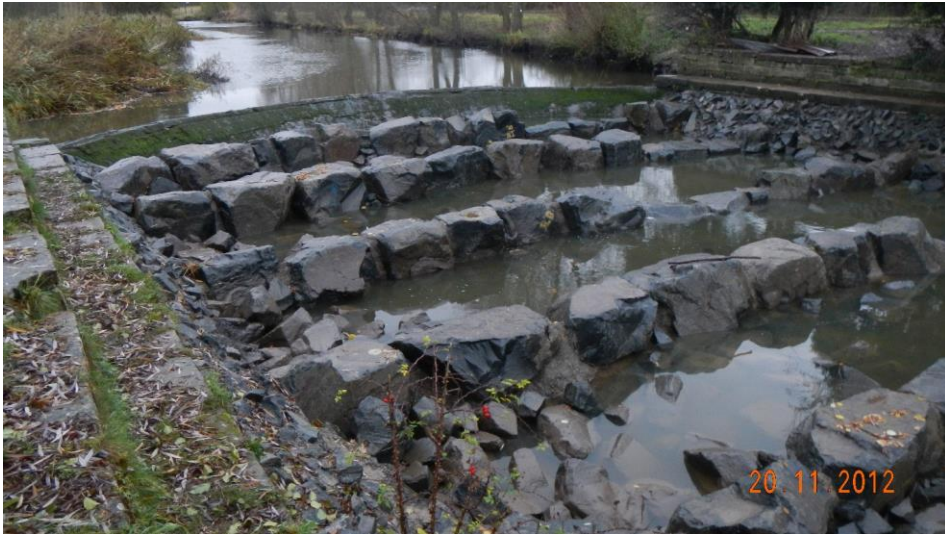
Photo 9 Rock ramp fish pass construction.
