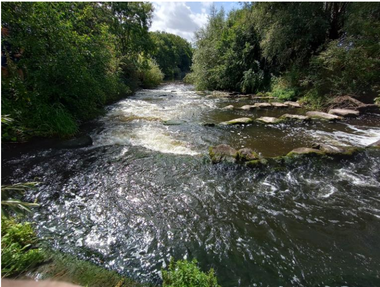
Photo 2 Rock-ramp fish pass at Arrow Mill weir, constructed in 2012 (see Appendix ).
