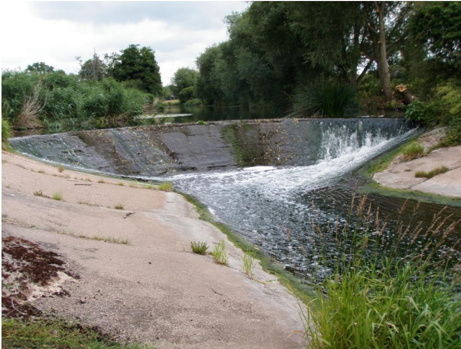
Photo 8 Weir above Arrow Mill before fish pass construction.
