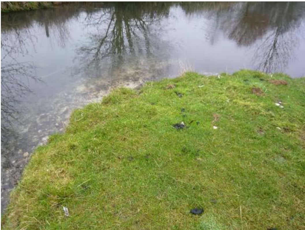
Imported chalk groyne designed to pinch the channel
