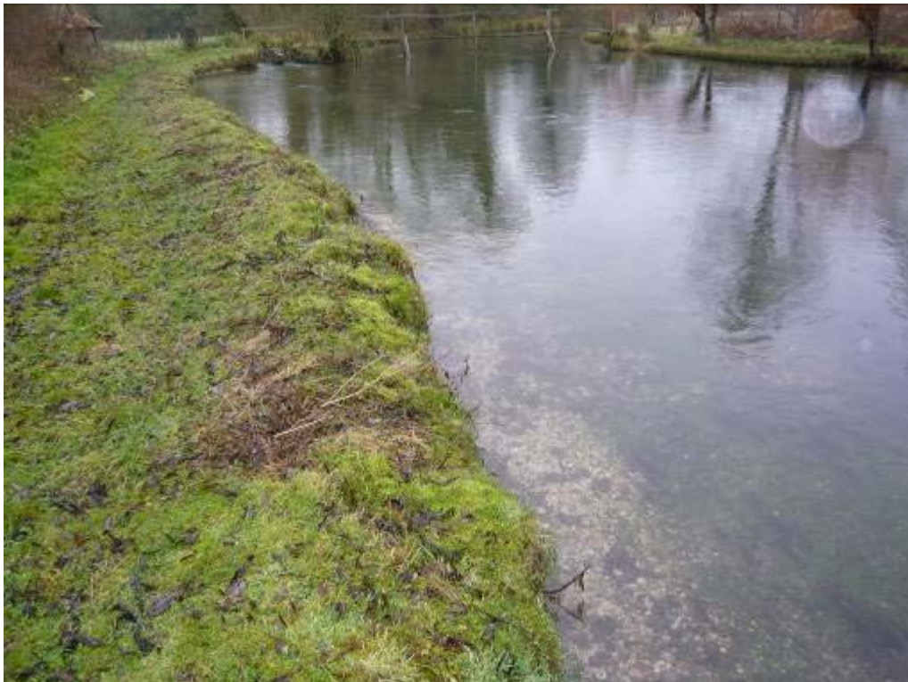
A biologically sterile margin. Man made banks without any sort of soft marginal fringe of emergent plants are often extremely vulnerable to bankside erosion.
