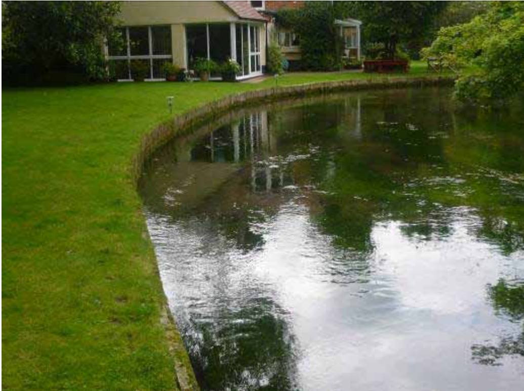
The LB adjacent to the garden is formally reveted with toe boarding. A fringe of marginal emergent plants would protect the bank and provide habitat
