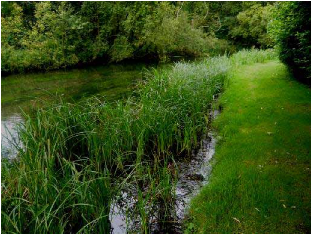
A new soft margin has been created by reveting the margin with faggot bundles. An excellent enhancement
