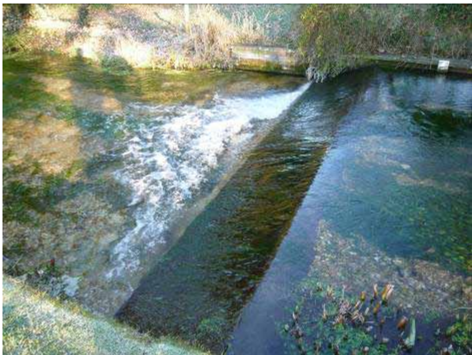
Flow gauging weir
