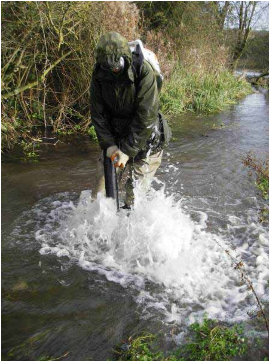
Cleaning gravels on a chalk stream with a back pack leaf blower
