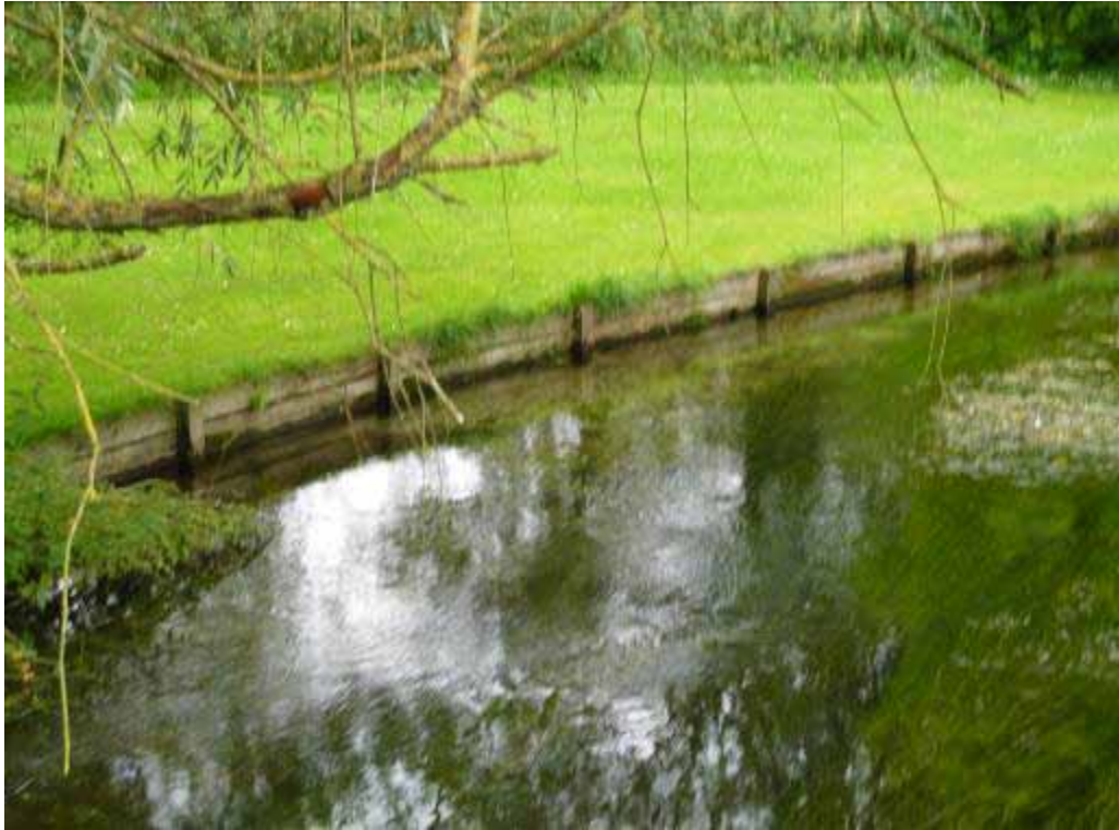
River bank revetted with wooden toe boards.
