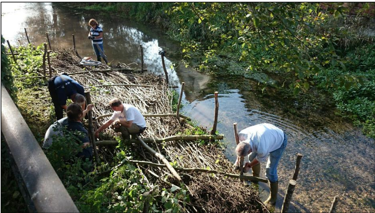
Figure 12: An example of a brushwood mattress installed on the River Allen at Witchampton Mill last summer
