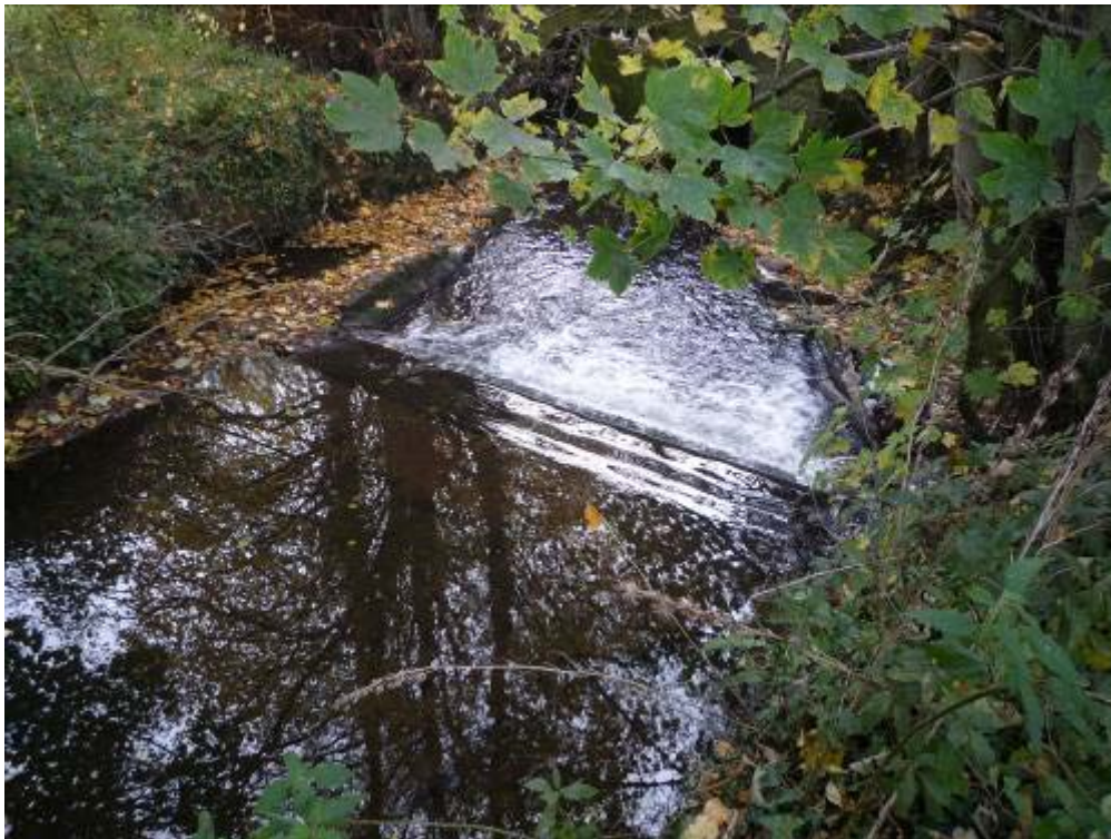
Small weir which could be improved by notching out the central section.
