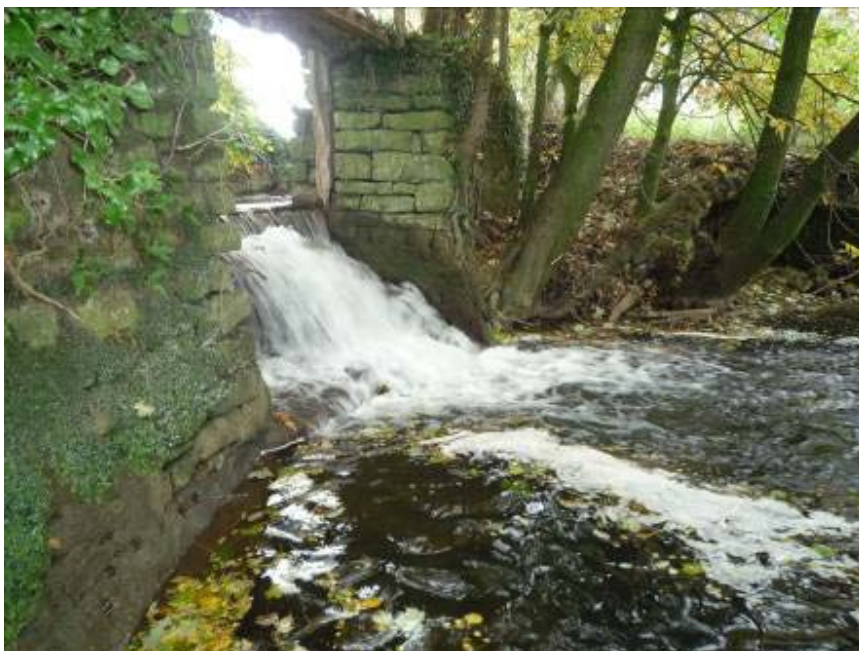
The main Silk Mill impoundment. This structure will fragment fish populations
