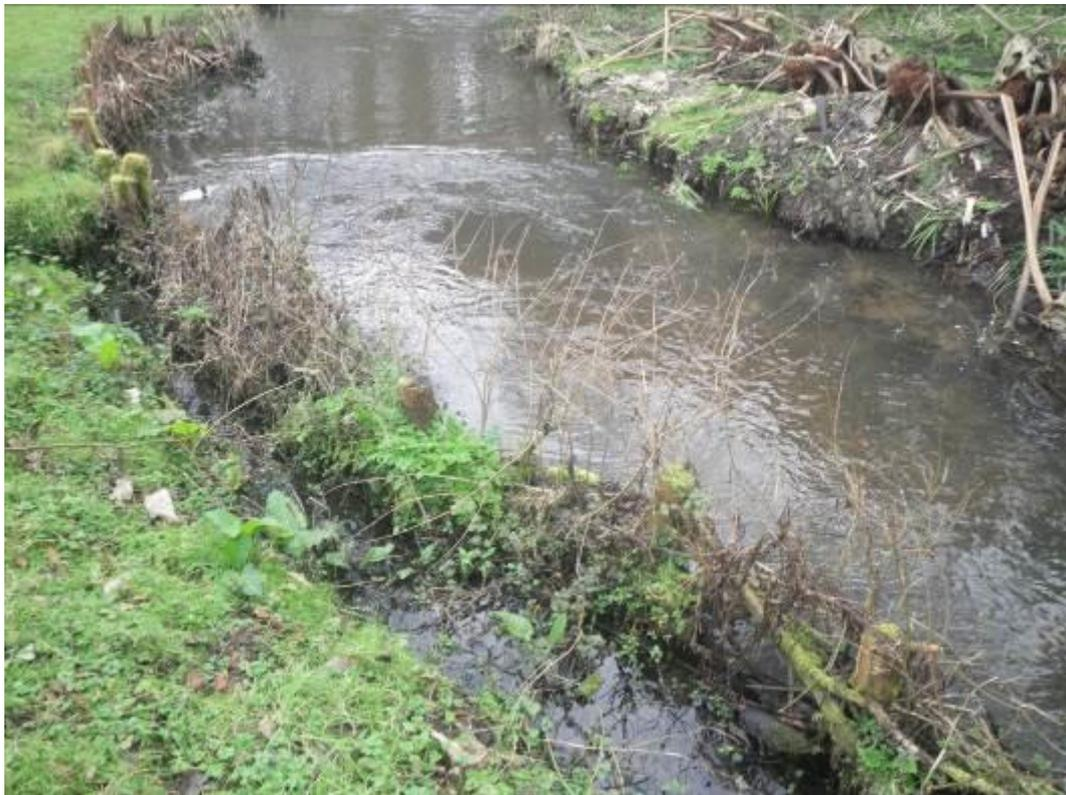
Photo 9. The live brushwood inserted into the outside of the bend will help to provide cover and protect the bank from erosive flow velocities.
