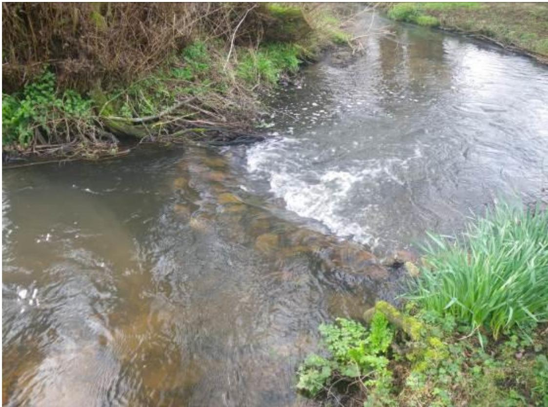
Photo 11. One of several low weirs designed to facilitate flow into the top lake.
