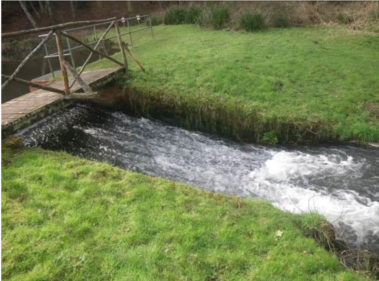
Photo 7. The dam and outlet structure of the bottom pond taking 100% of the flow of the Tillingbourne and completely blocking access for migrating wild fish.
