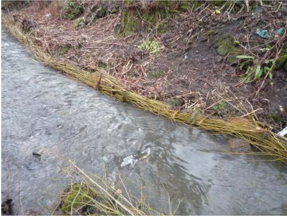
An excellent spawning and nursery stream where the margins have been defended with live willow weave.
