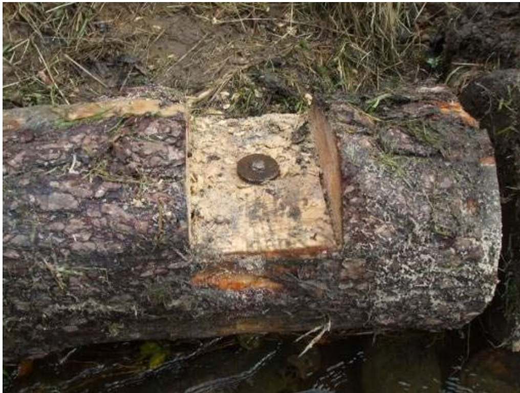
A piece of LWD secured to a stream bed with 2m of 22mm steel reinforcing bar with a welded steel retaining washer
