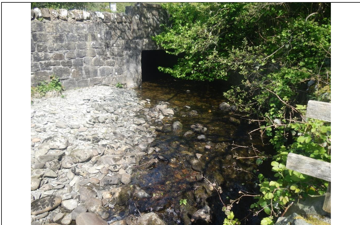
Figure 25. What appeared to be free passage beneath the road bridge.
