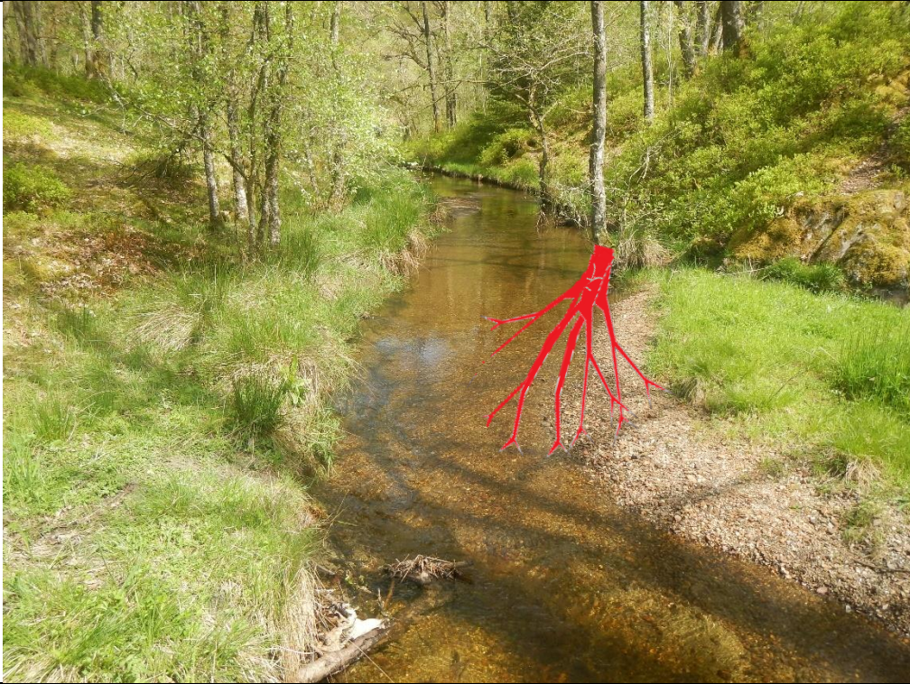
Figure 21. The natural sinuosity of the channel and fish cover could be enhanced here with the addition of woody material. The bankside trees provide a great anchor point for Pinned Woody Material (red diagram).
