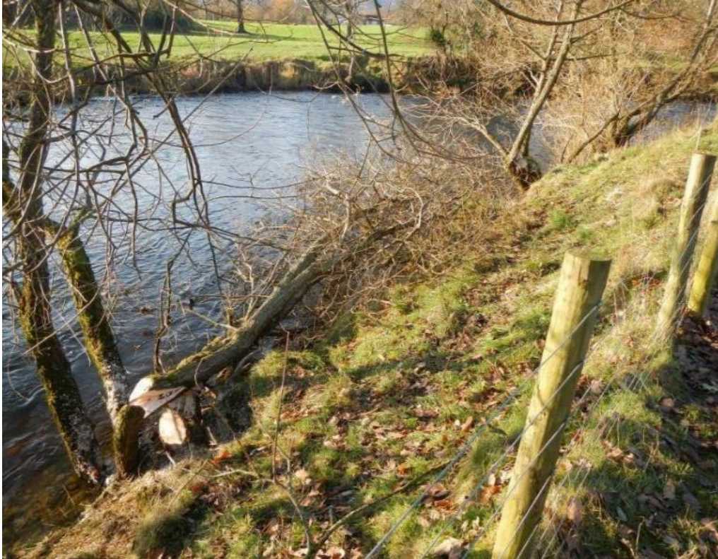
Figure 40. Willow hinged into the river margin to increase cover and structure. The method involves cutting part way through the stem, quickly through the first two thirds, then continuing until it collapses or can be pushed down over the river. The depth of the cut should be limited to only that which is required to bend the stem over, as this will maintain maximum size and strength of the hinge and the health of the tree/shrub.
