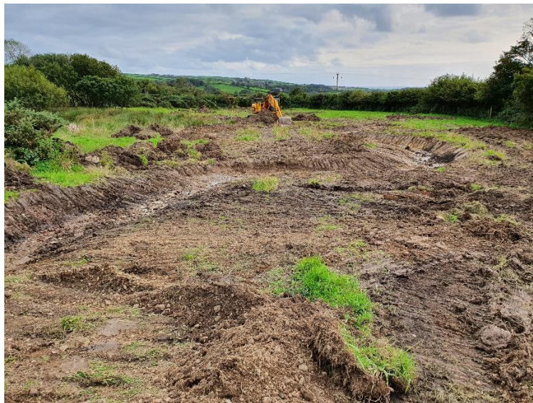
Black Beck – during restoration / channel excavation.
