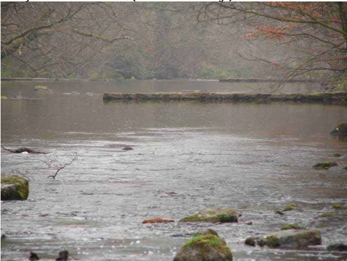
Two dams d/s Allensford Bridge, which can be seen to be having an effect on flows upstream (silt-trap)
