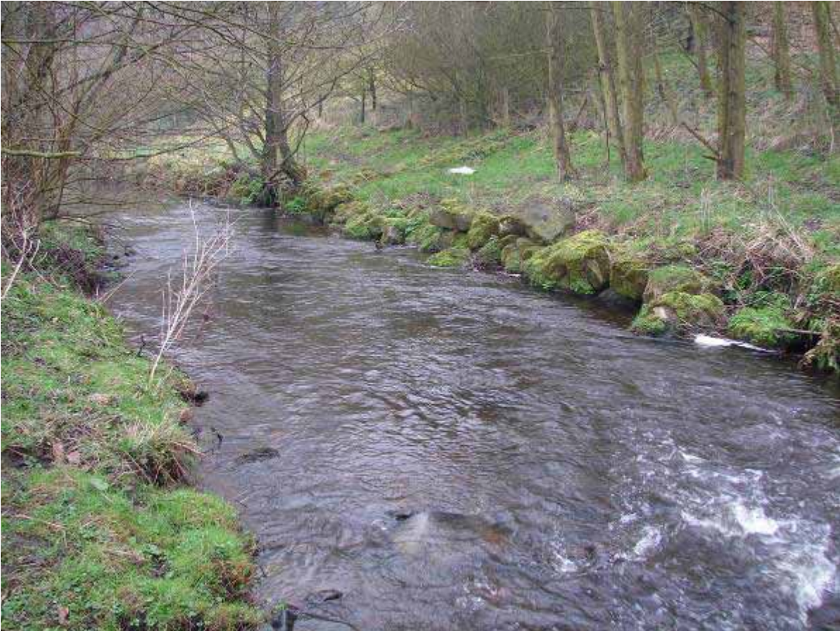
Stone revetment on RHB
