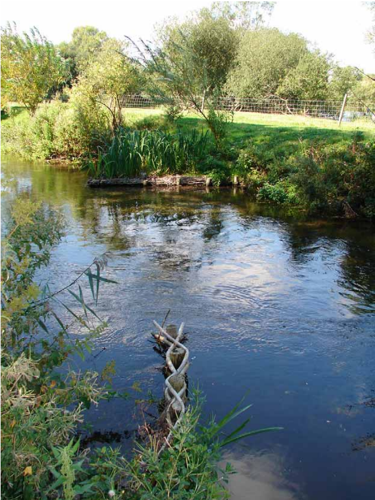
Introduction of single u/s 'natural' deflectors (single, near bank and triangular' far bank) on the Wylle in Wiltshire formed a chicané, sending flow from one bank to another. Note set just above summer water levels.
