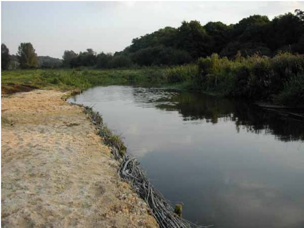
Installation of new bank using faggots and chalk backfill on the River Wensum, Norfolk
