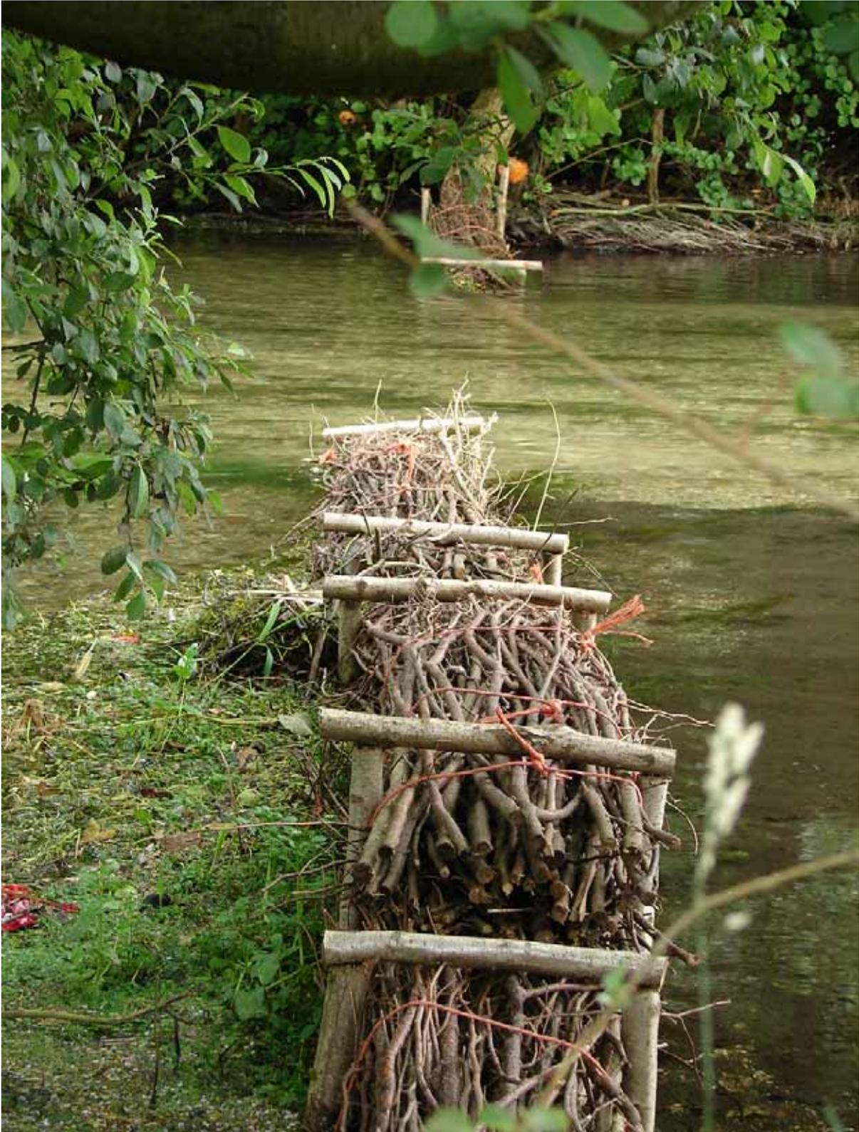
Picture 4) – Recently installed paired faggot deflectors. Note silt deposition and scoured gravel d/s of faggots. Note 90-degree position.
