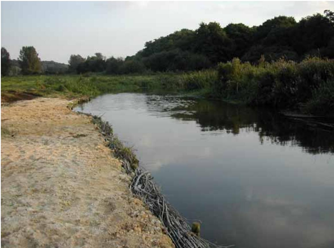
**Picture 6) Installation of new bank using faggots and chalk backfill on the River Wensum, Norfolk**
