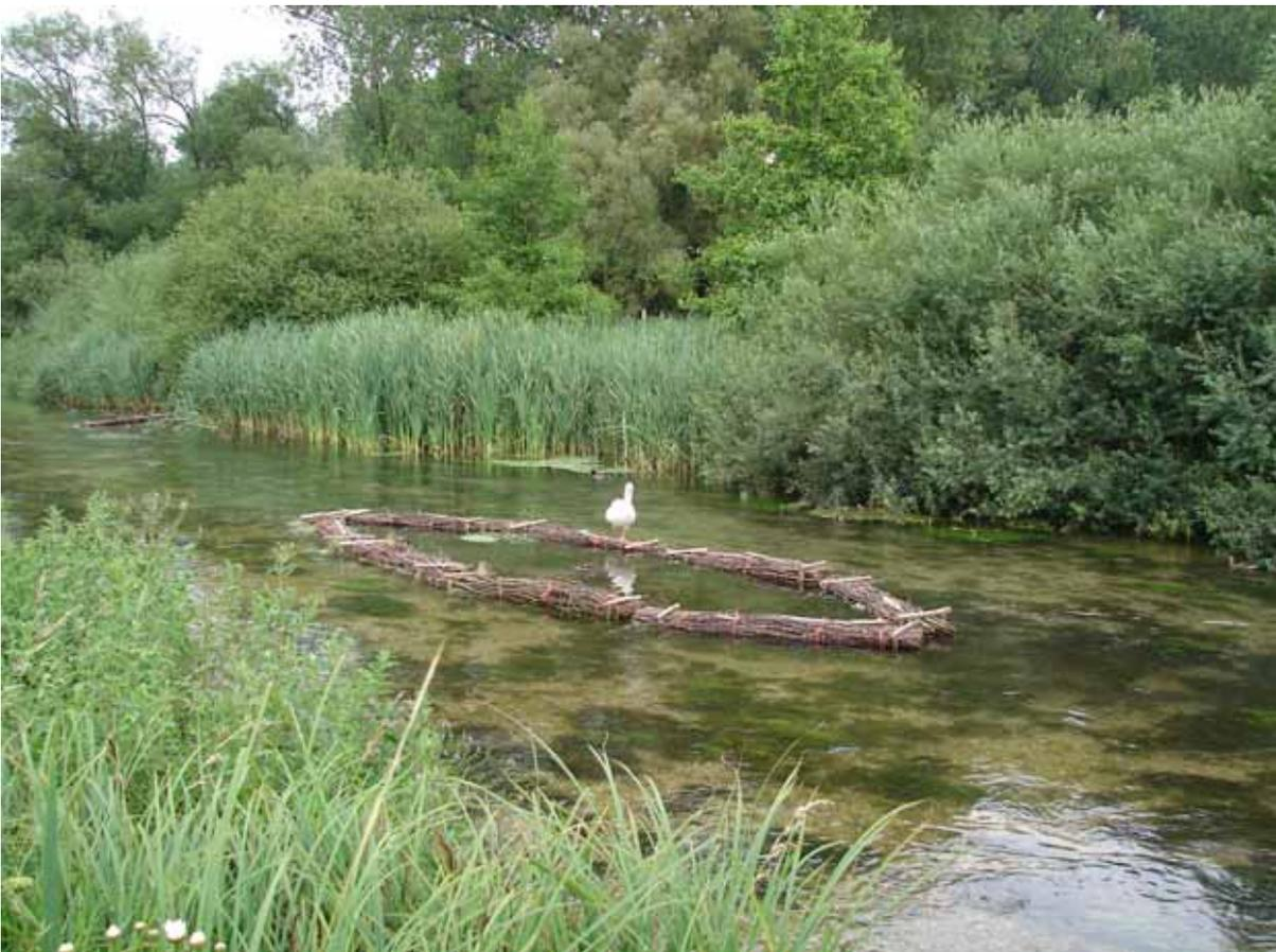
Picture 3) recently installed 'faggot Island'
