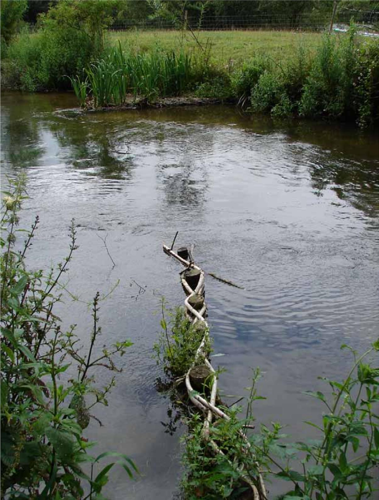
**Picture 7) Introduction of single u/s 'natural' deflectors (single, near bank and triangular' far bank) on the Wylde in Wiltshire formed a chicane, sending flow from one bank to another. Note set just above summer water levels.**
