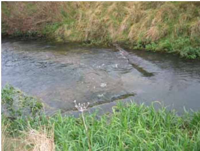
Paired upstream facing wooden groynes. Note how ends are keyed into the bank in order to prevent erosion.
