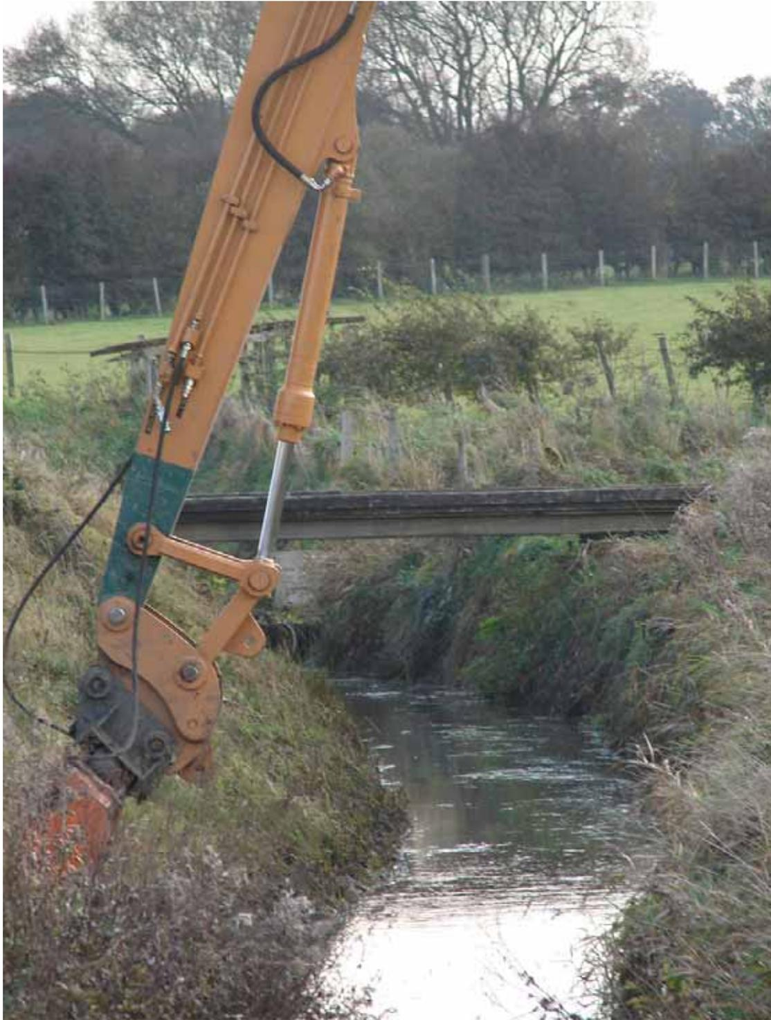
**Close-up of EA 'slubbing-out' operation. Note removal of vegetation from toe of the dyke. This is important habitat for water voles for foraging, predator avoidance and latrine requirements.**
