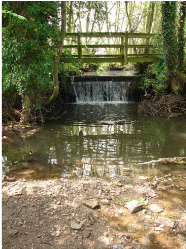
E) Pump House Weir
